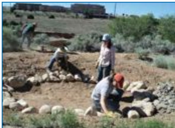
Volunteers building bio-retention structures for storm-water run off
