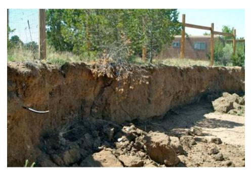
Photo 17: Arroyo de los Chamisos eroding the land close to a property line and exposing cables. Source: Keely Jackson Kennemore, SFWA 2012.
