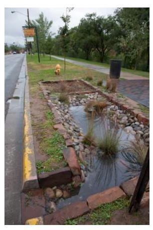
Photo 15: Curb cut with infiltration basin along West Alameda Street in Santa Fe.
