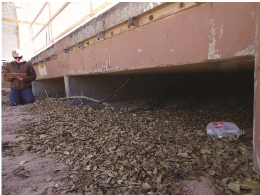
Segment E / Paseo de Peralta box filled with sand, Arroyo Rosario, 2016.
