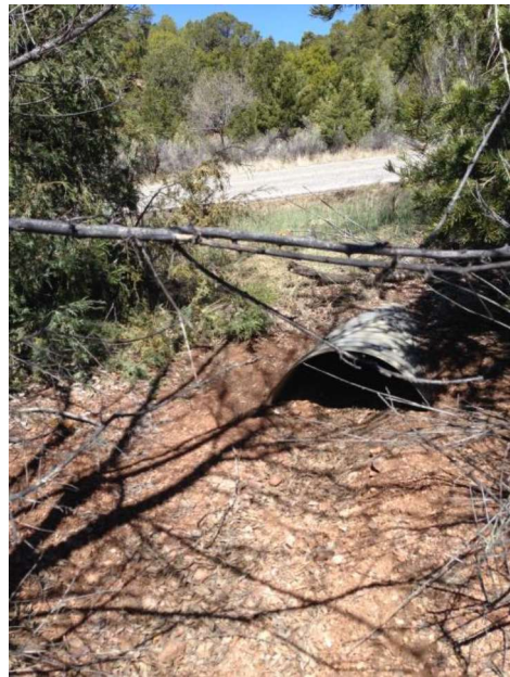
Segment A/Obstructed culvert, Arroyo Ancha, 2016
