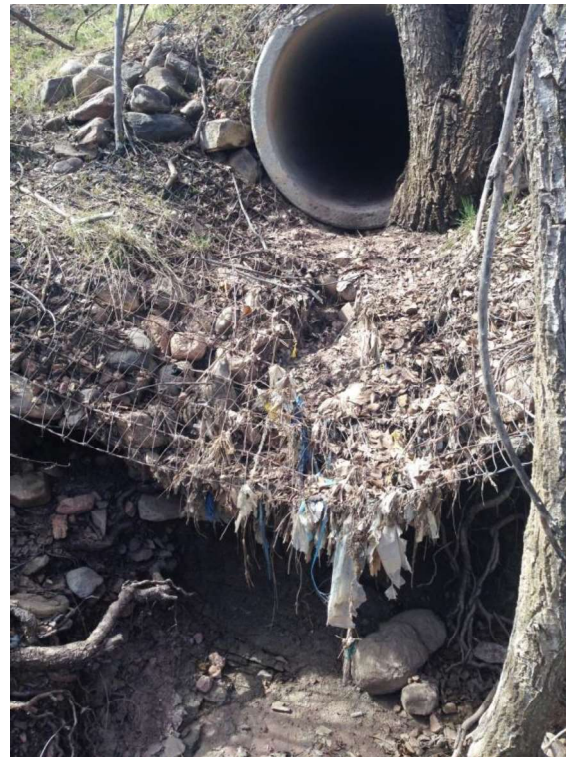
Undercut rip rap 2012 and trash below a culvert off Camino Cabra vs 2016, Arroyo Cabra, 2016
