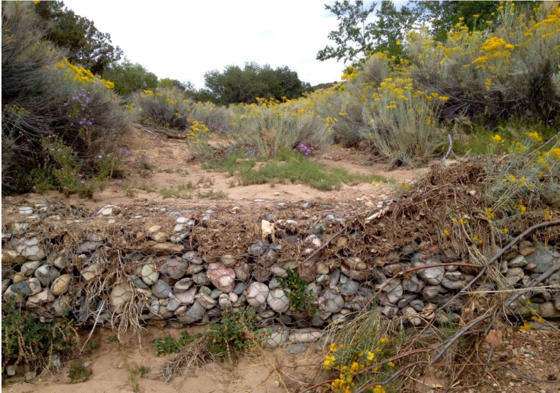
Segment B/ Gabion check dam in 2012, Arroyo Piedra.
