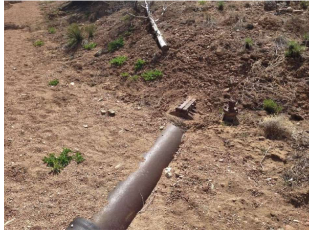
Segment A/ Comparison of exposed iron pipe. Left 2016 condition/ Right 2012 condition, Arroyo Piedra, 2016.
