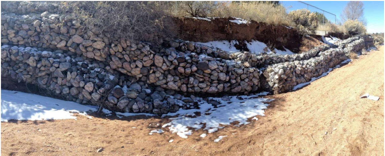
Segment C/Gabion walls coming off arroyo bank, 2016.
