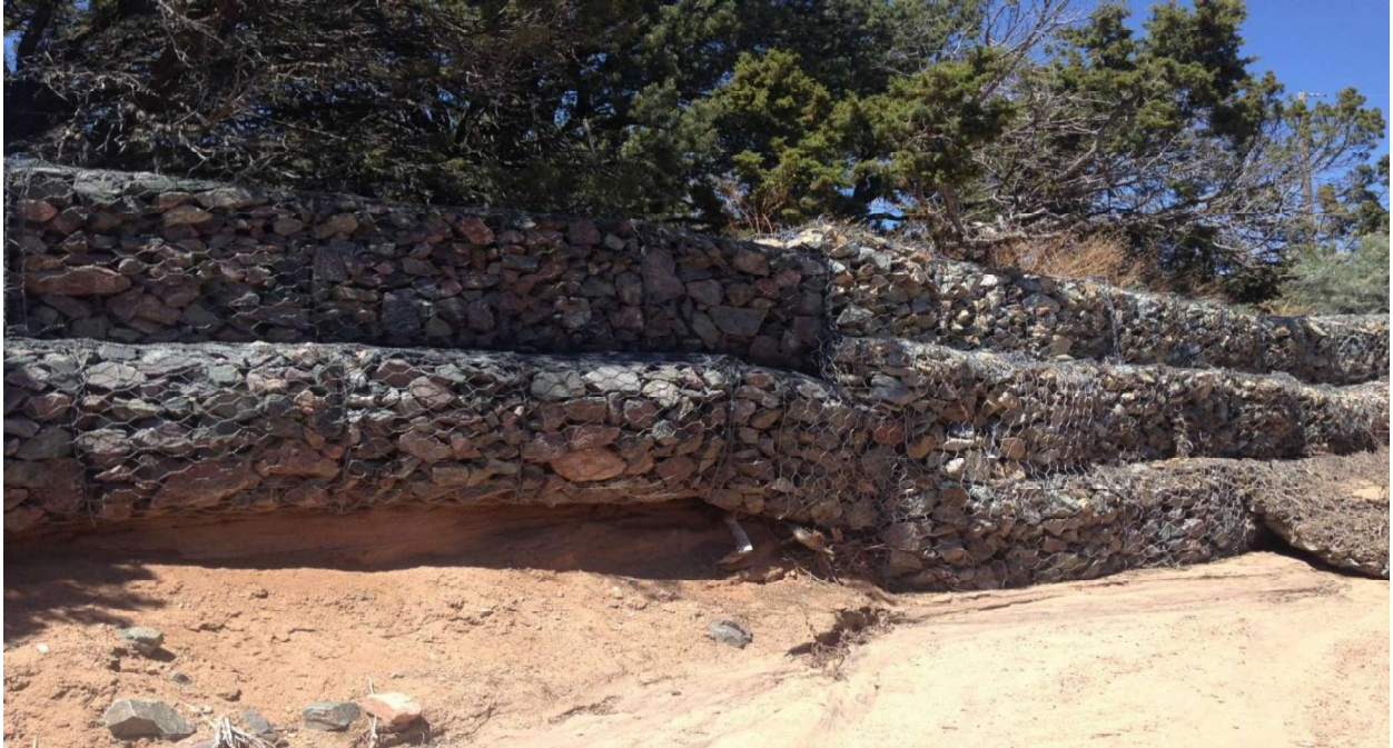
Segment B/Erosion below gabion walls, Arroyo Cloudstone, 2016.
