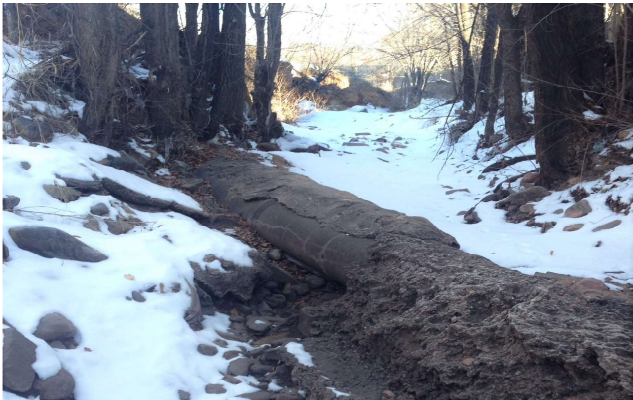
Segment C/Cracked concrete pipeline, Lower Arroyo Pinos, 2016.
