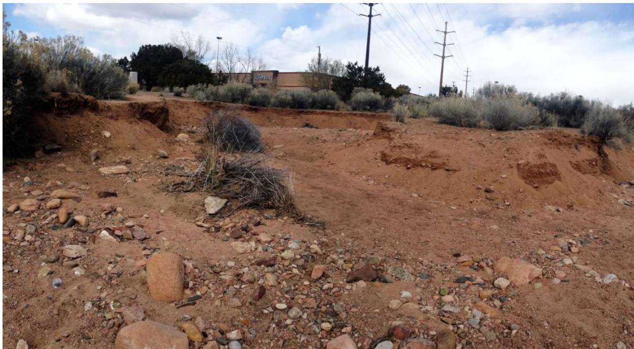
Segment H/Side channel bypasses gabion wall, Arroyo de los Chamisos, 2016.
