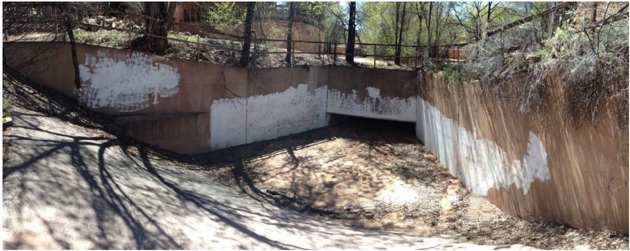
Segment B/ Sediment level rises beneath box culvert E. Alameda St. in Arroyo Ancha, 2016
