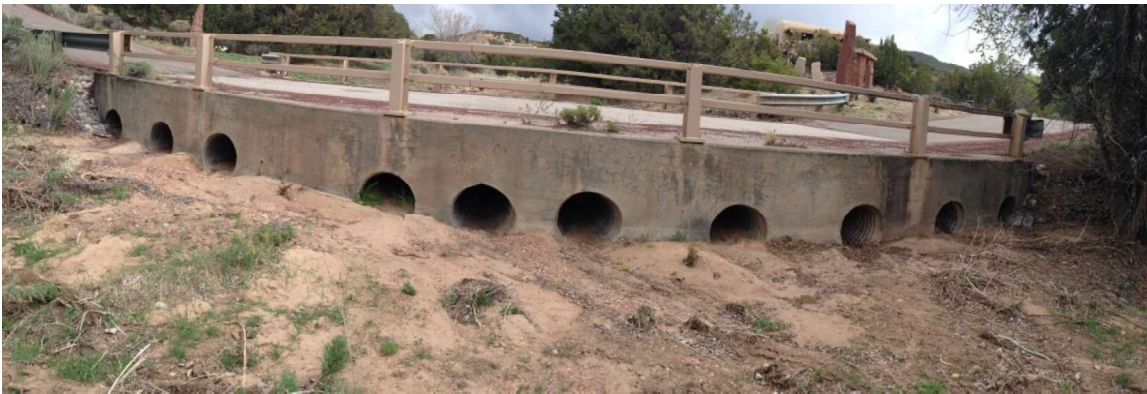
Segment B/ Downstream side of restricted culverts , Arroyo Piedra, 2016.
