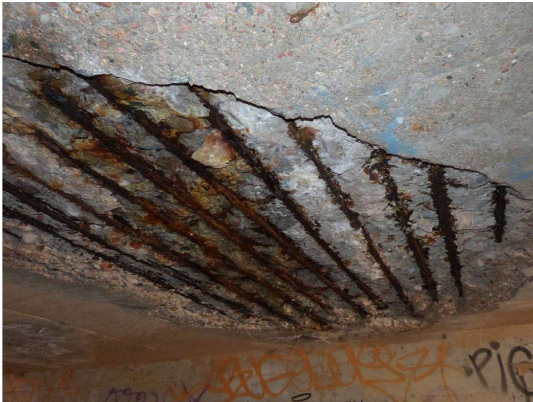
Segment B/Underside of concrete damage, Old Taos Bridge Arroyo Mascaras ,2016.
