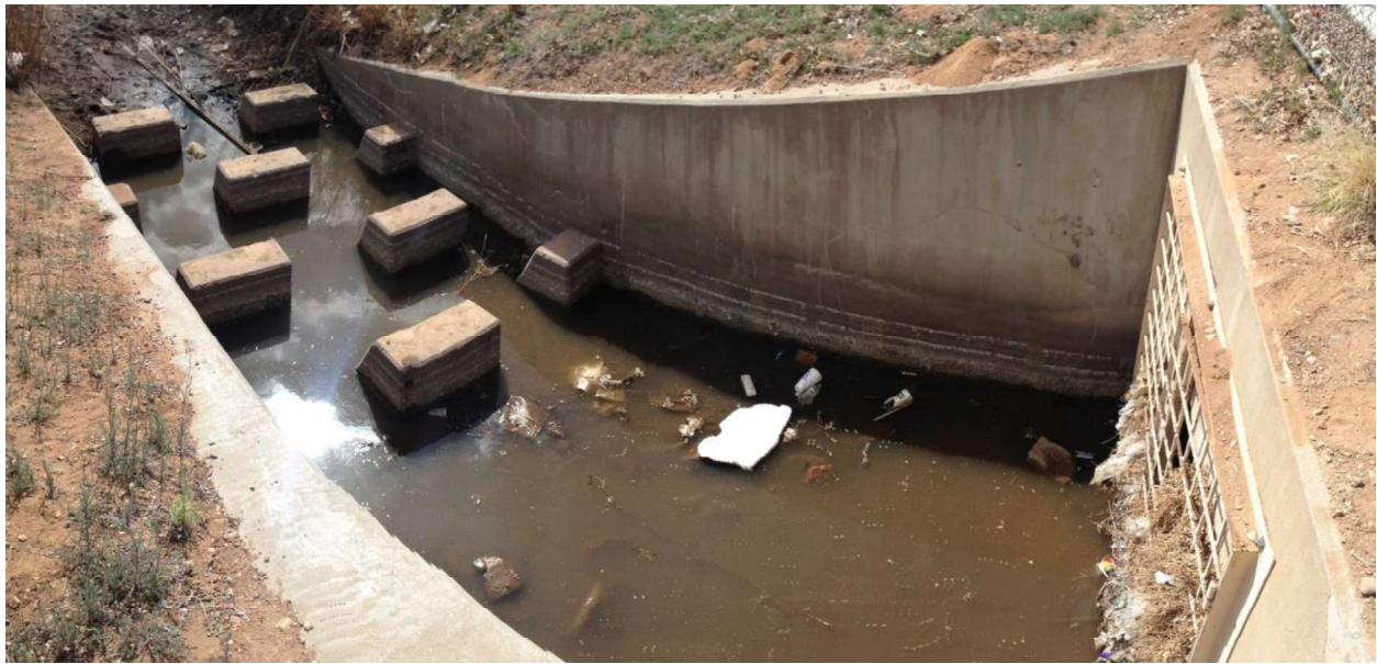
Segment H/Culvert obstructed with trash, Arroyo de los Chamisos, 2016.
