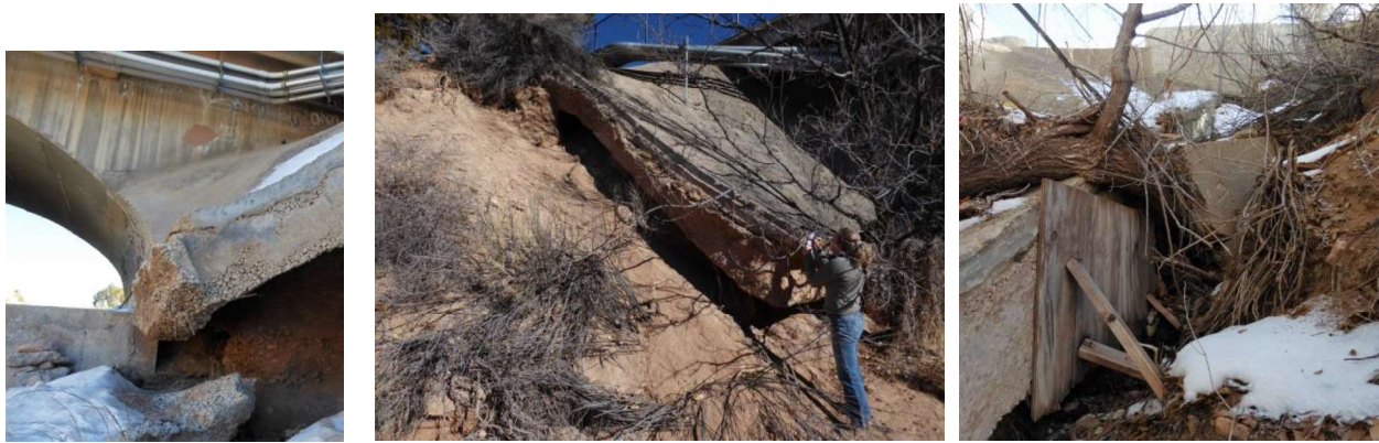
Segment D/ Vo-Tech Bridges with examples of eroding banks and footings, Arroyo Chamisos, 2016.
