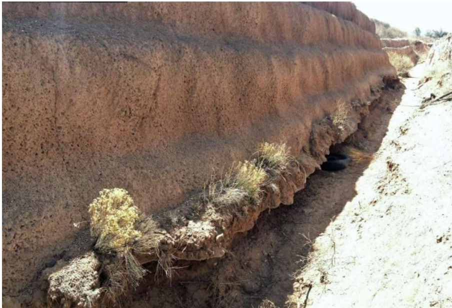
Segment B/Two views of engineered walls made of tire and adobe with undercutting, Arroyo Torreon, 2016.
