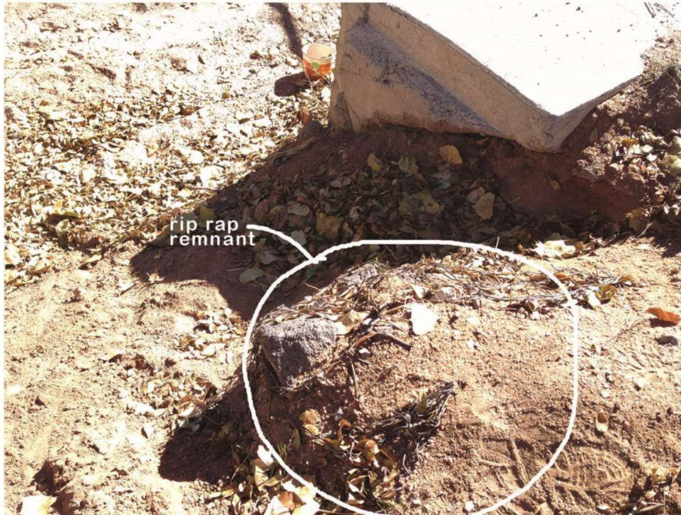
Figure 2 Segment E / Birds eye view of eroded west bank and culvert shoulder, 2016
