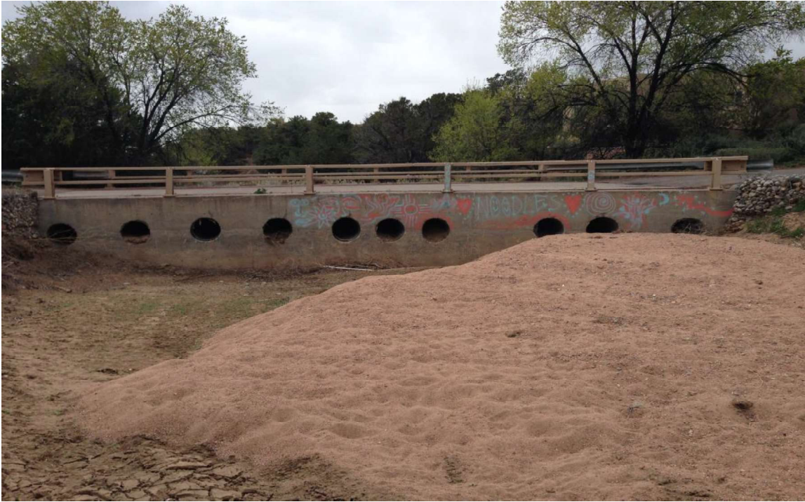
Segment B/ Upstream side of restricted culverts with sediment displacement , Arroyo Piedra, 2016.
