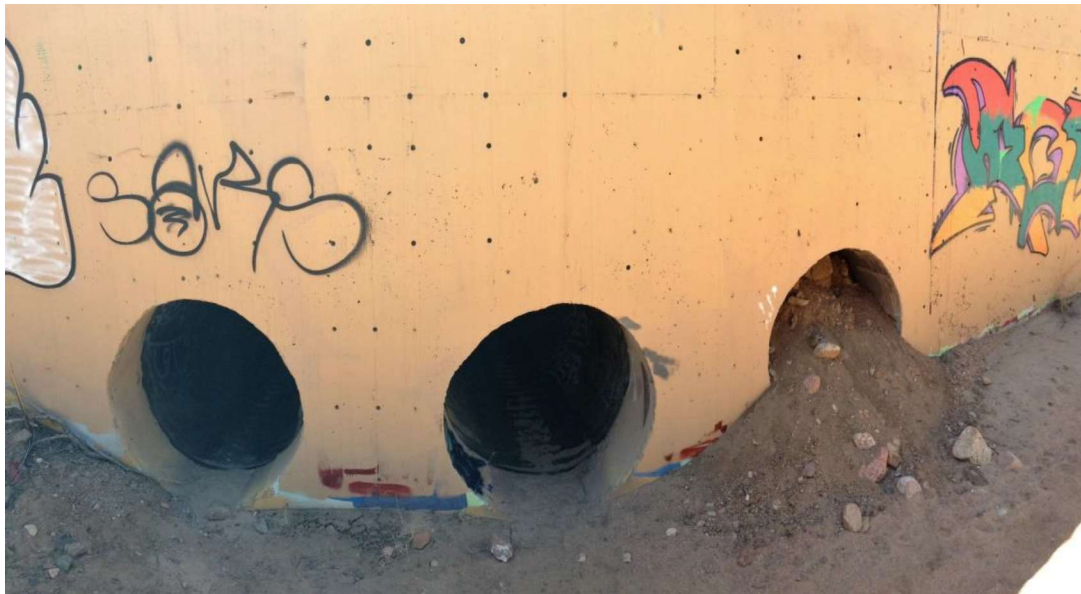
Segment A/ Obstructed culvert, Old Pecos Trail, Upper Arroyo Pinos North, 2016
