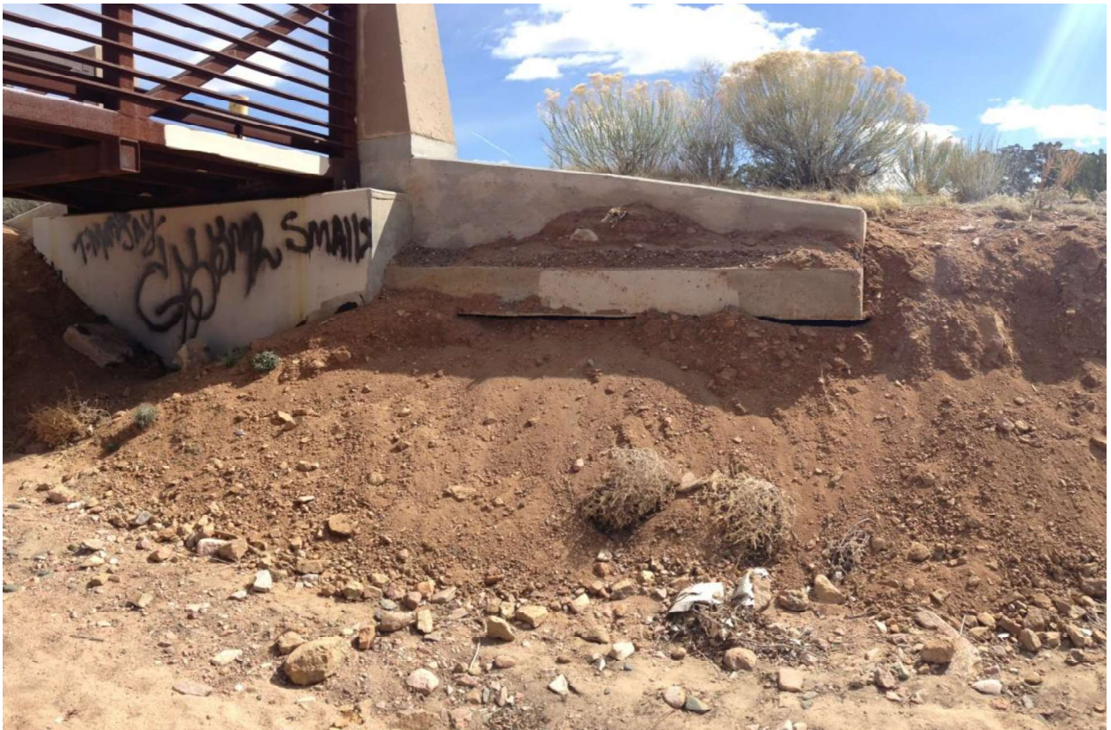
Segment H/Pedestrian bridge with exposed footing, Arroyo de los Chamisos, 2016.
