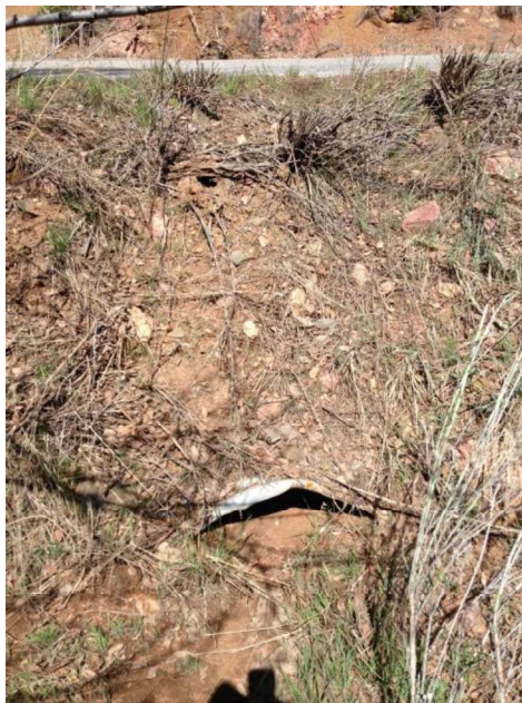
Segment A/Obstructed culvert, Arroyo Ancha, 2016
