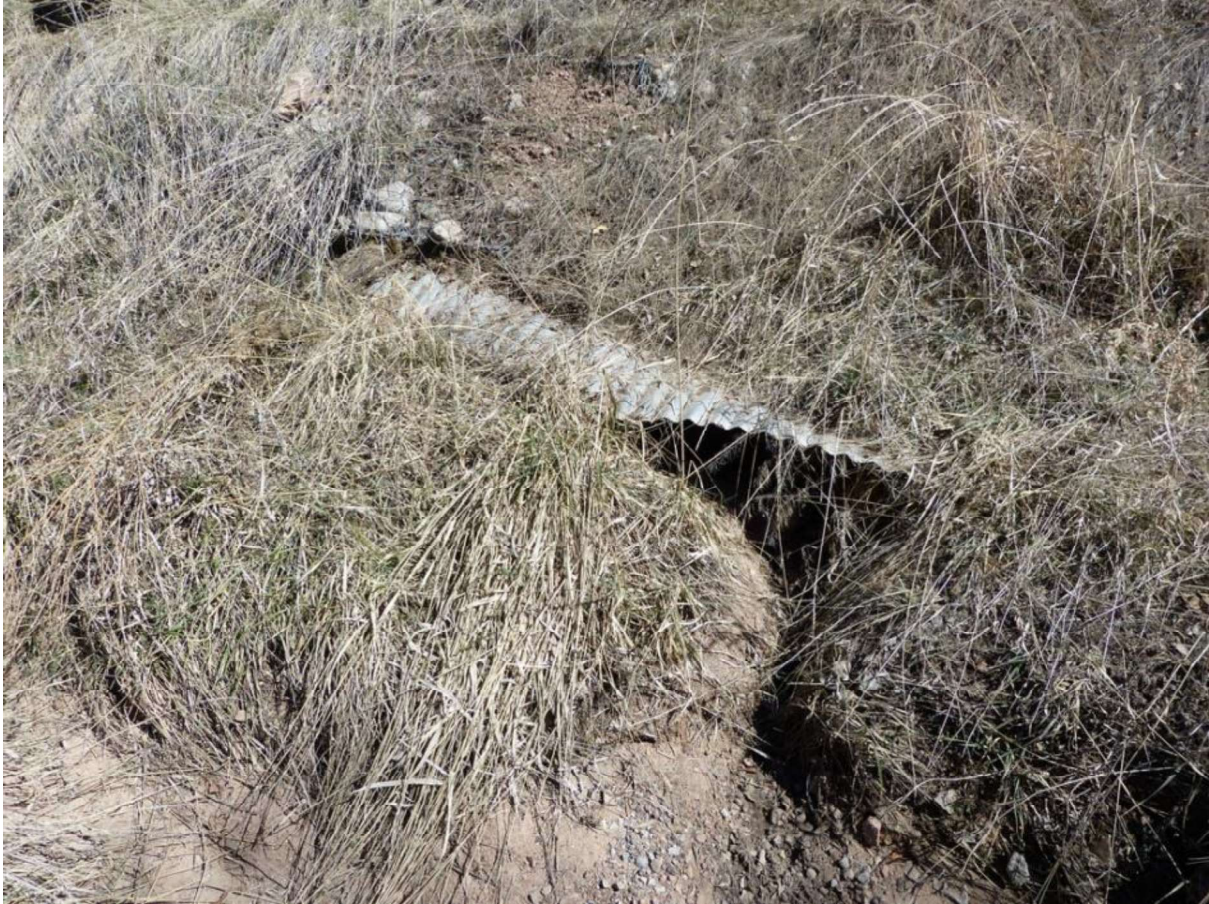
Silt clogged culvert in the Arroyo Saiz, 2016.
