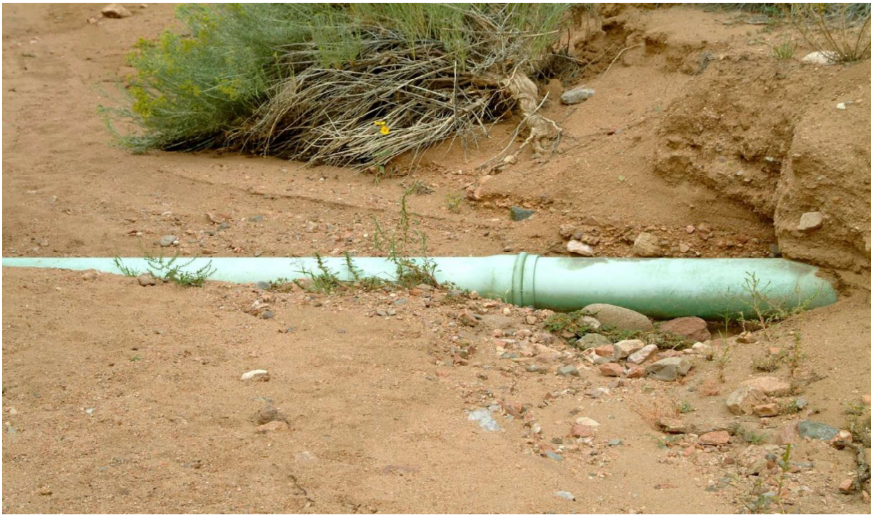
Segment G/A partially exposed pipeline, Arroyo en Medio, 2012
