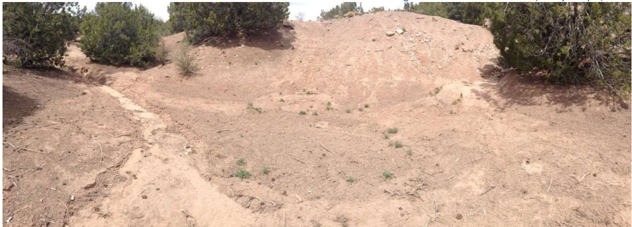
Example of storm water bypassing upper catchment basin as it enters the lower basin, Arroyo Nopal, 2016.
