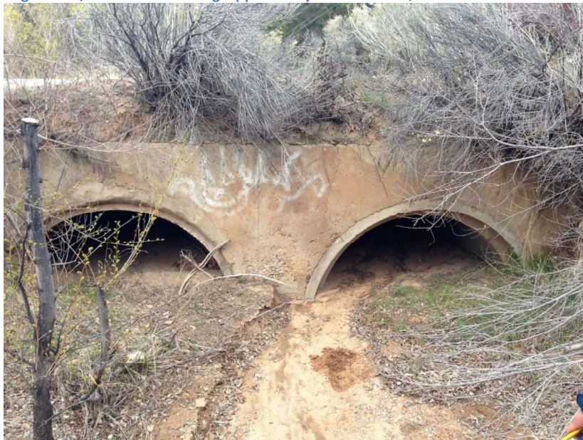
Segment B /Obstructed culvert Upper Arroyo Pinos South, 2016.
