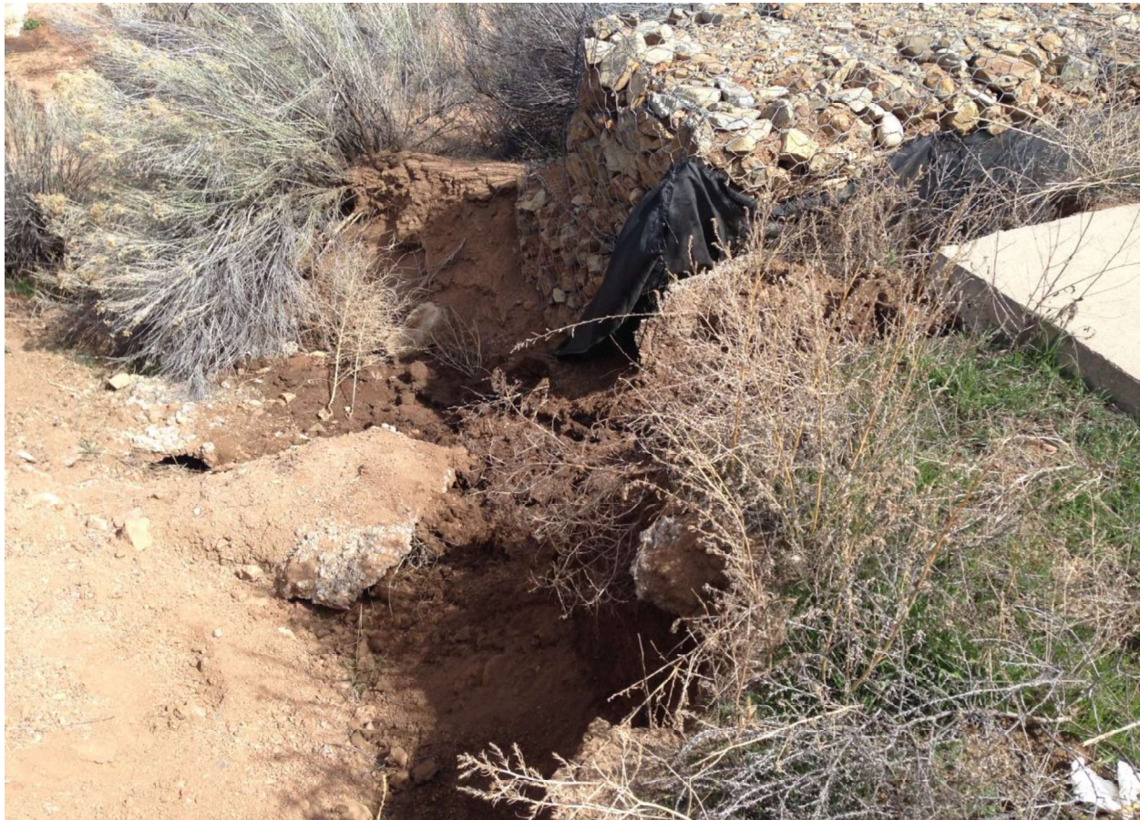
Segment B/ Erosion below sewer outlet, Arroyo Chaparral,2016.
