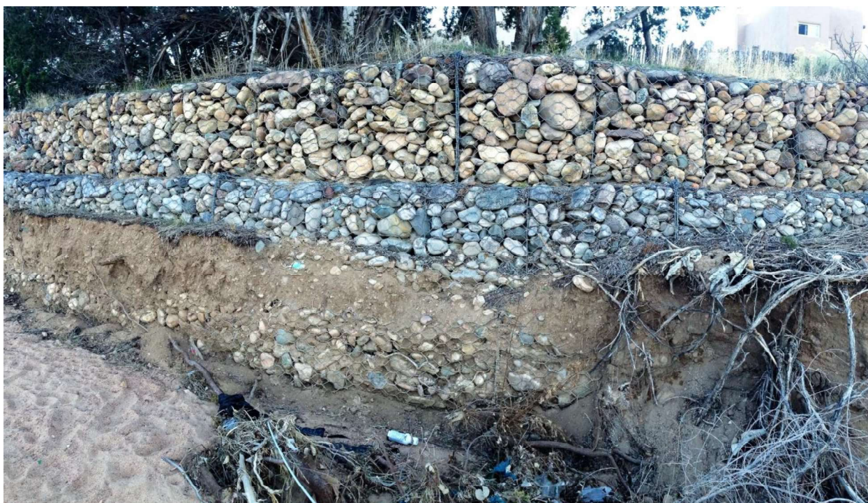
Segment H/ Illustration of sediment fluctuations. Sediment levels remain intact against gabion wall at far right of photo while left and center sediment no longer exists, Arroyo de los Chamisos, 2016.
