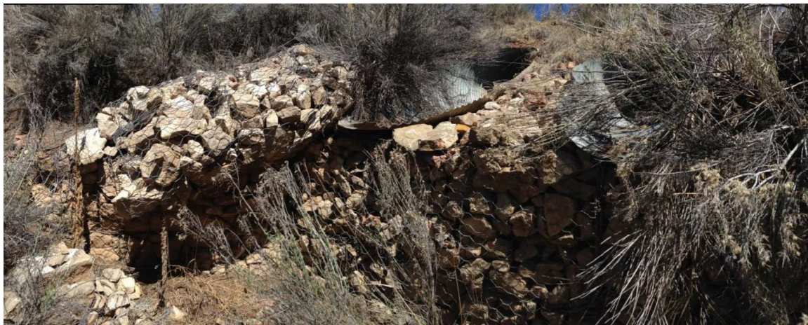
Segment A/Gabion askew, Arroyo Ancha, 2016.
