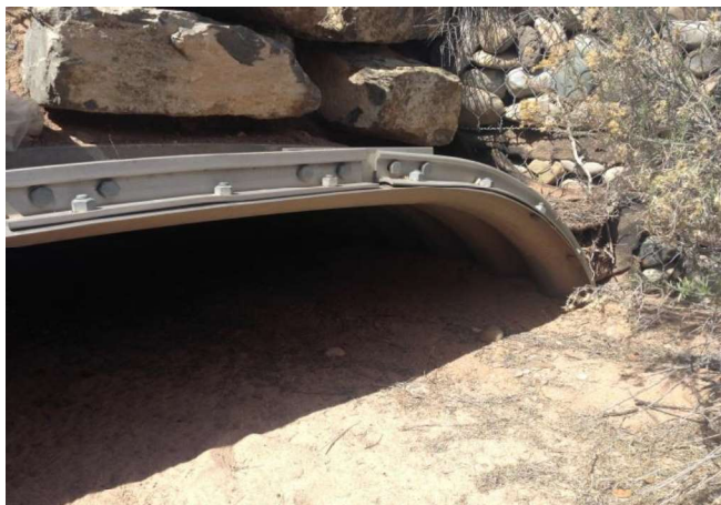
Segment A/Silt trapped in culvert, Arroyo Torreon, 2016.
