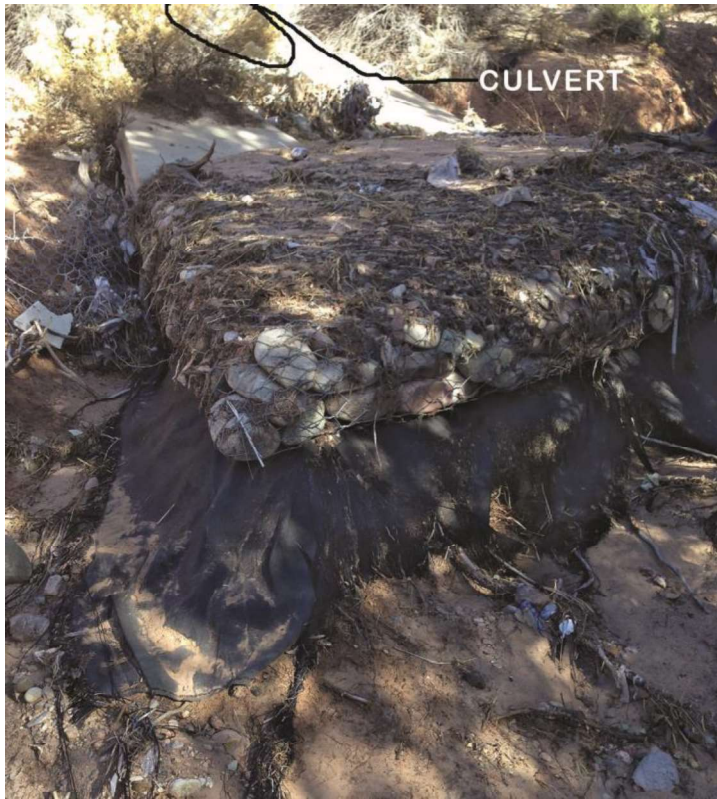
Segment A/ Erosion beneath rip rap mat, Arroyo Rosario, 2016.
