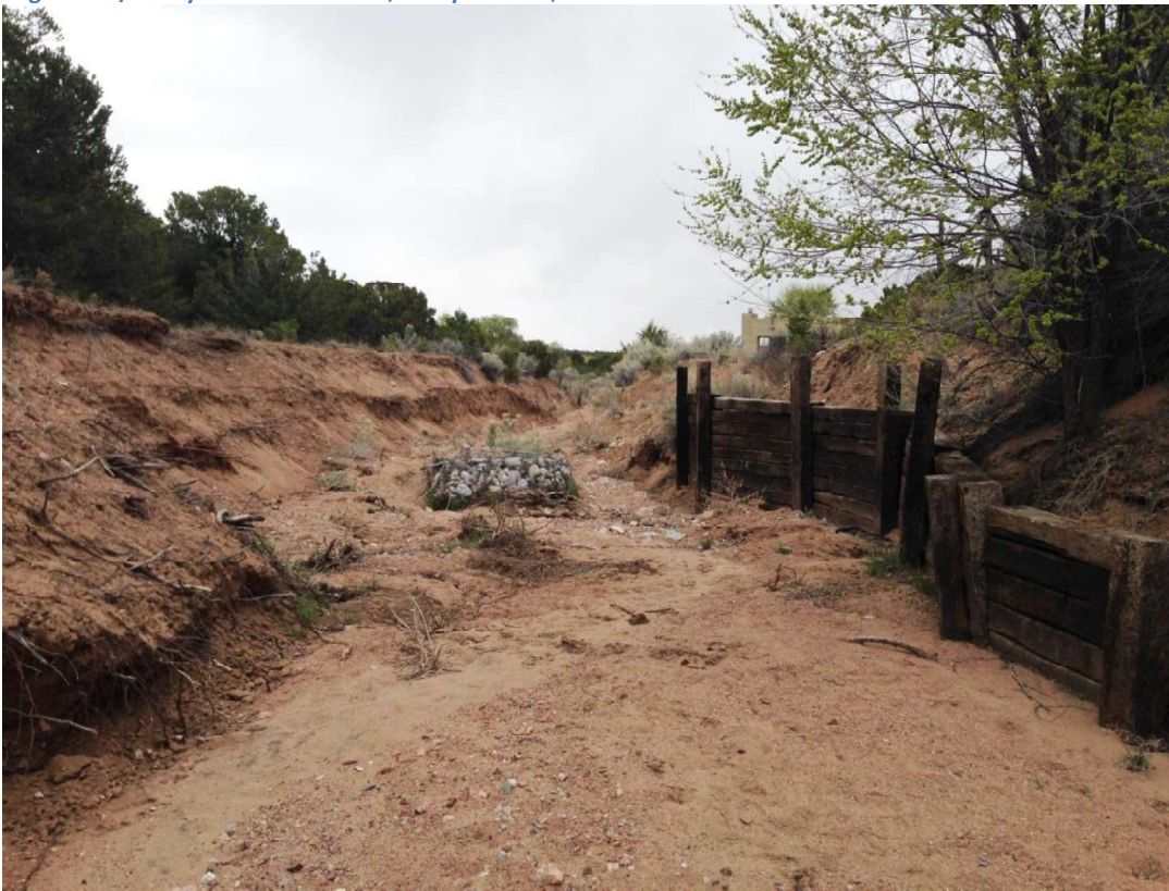
Segment B/ Retaining wall and gabion basket added to arroyo channel, Arroyo Piedra, 2016
