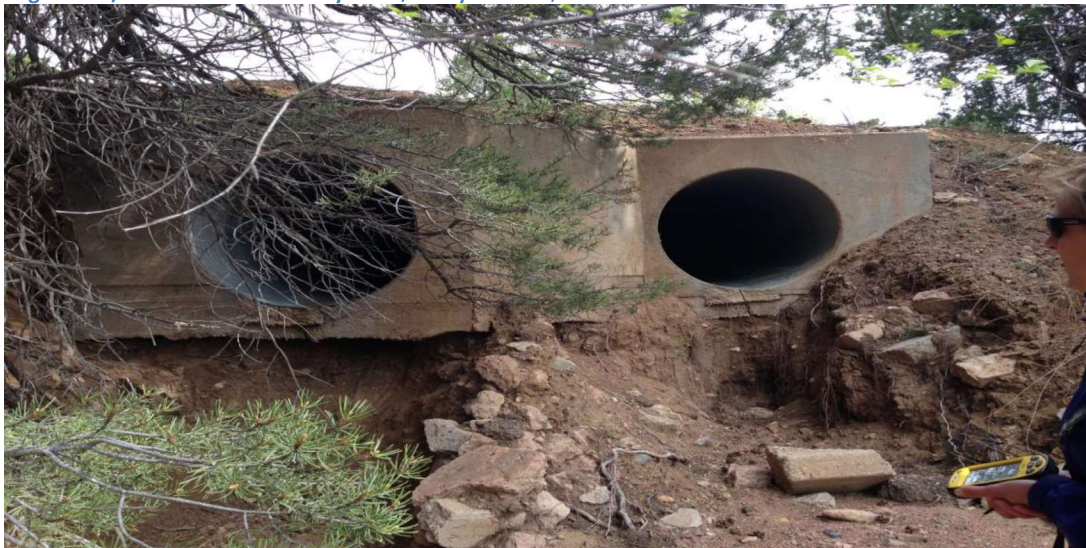
Segment B/Bank deterioration below culverts, Arroyo Piedra, 2016.
