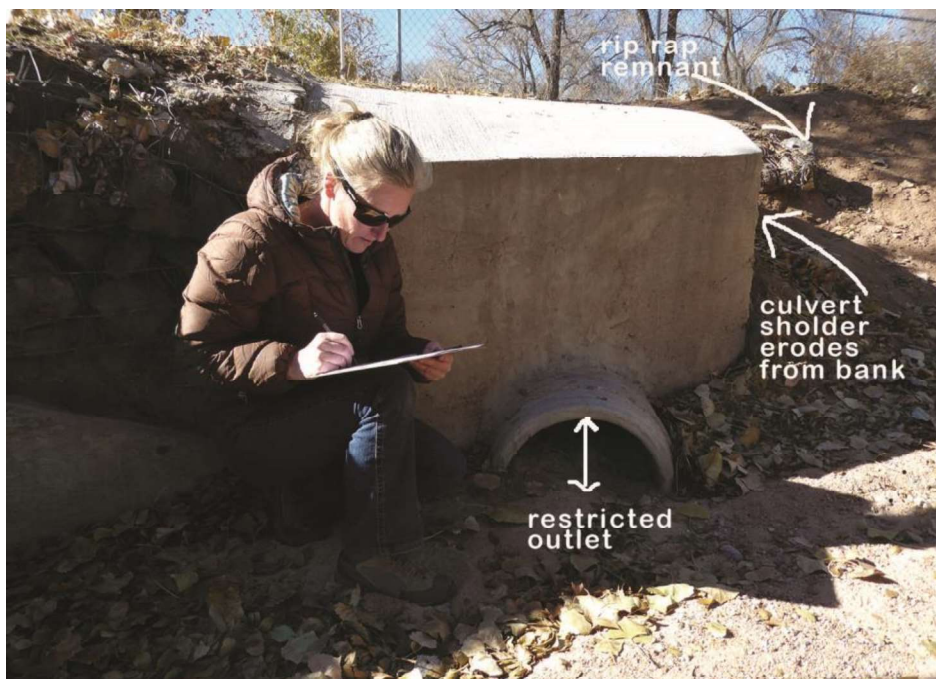
Figure 1 Segment E/ View of restricted outlet and eroded west bank,2016
