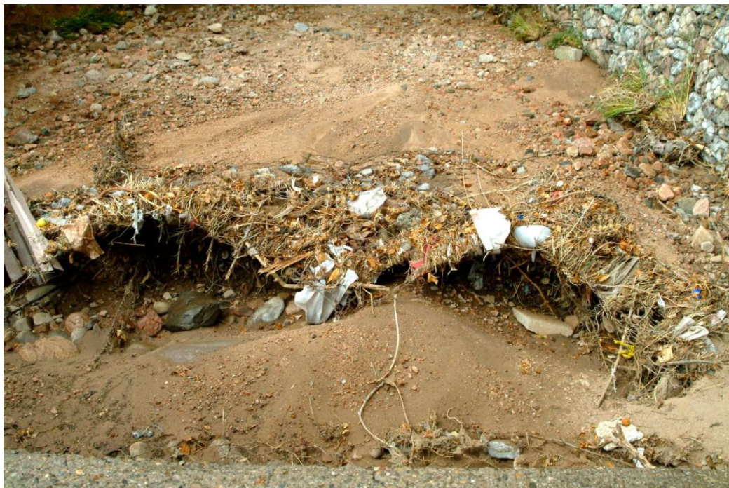
Segment D/ Damaged rip rap mat 2012, Lower Arroyo Pinos.
