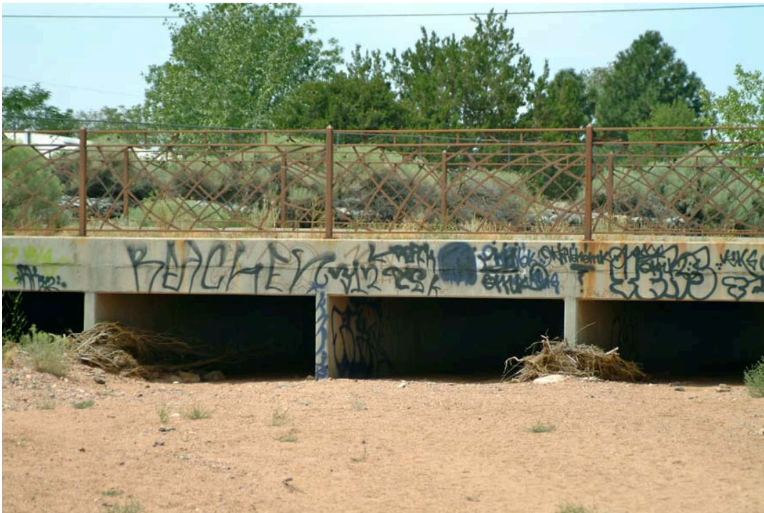
High levels of sediment under Botolph Bridge in Segment C of Arroyo de los Chamisos.
