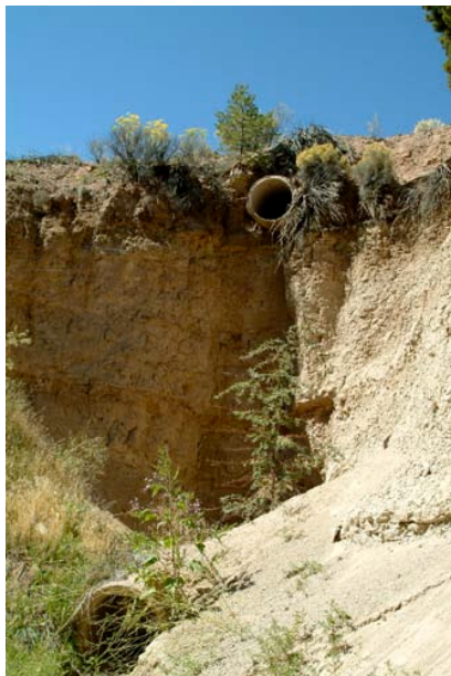
Damaged culverts, Arroyo Piedra West, Segment B.
