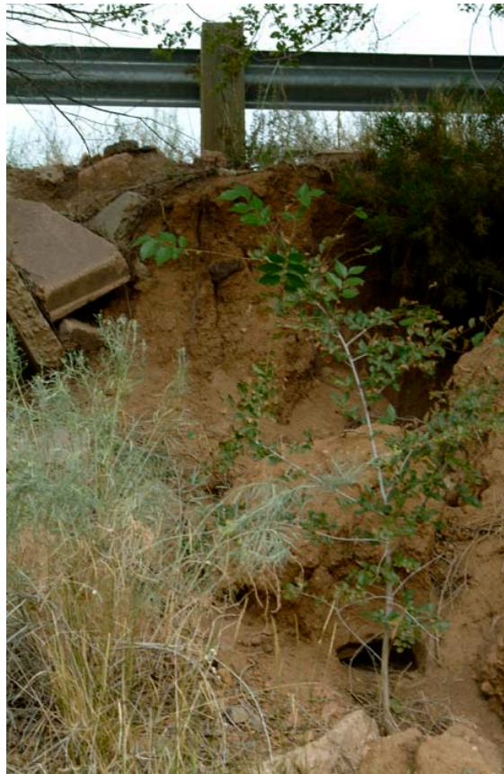
Erosion of shoulder off Old Pecos Trail Road, Segment C.
