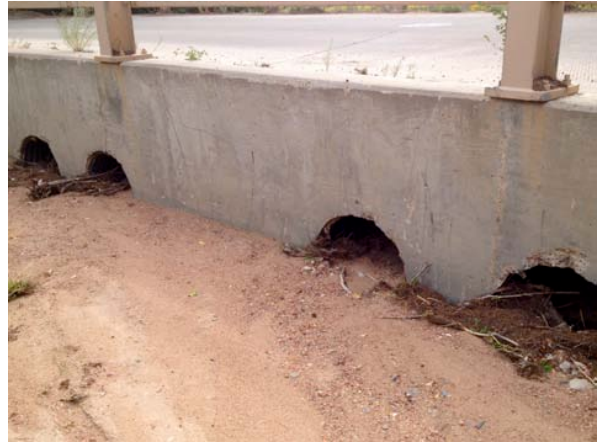
Obstructed culverts crossing Arroyo Piedra East, Segment A.
