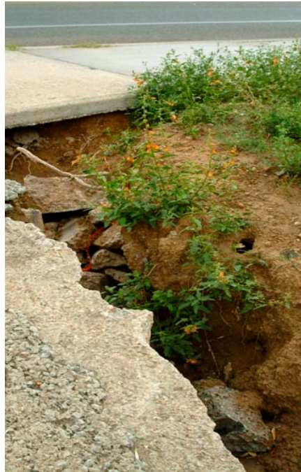
Erosion at Camino Carlos Rey Bridge, Lower Arroyo Pinos, Segment D.
