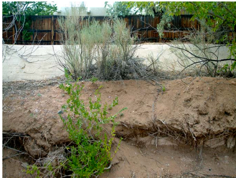
Severe bank erosion encroaches on the Arroyo de la Chamisos Trail creating hazardous conditions in Segment E.
