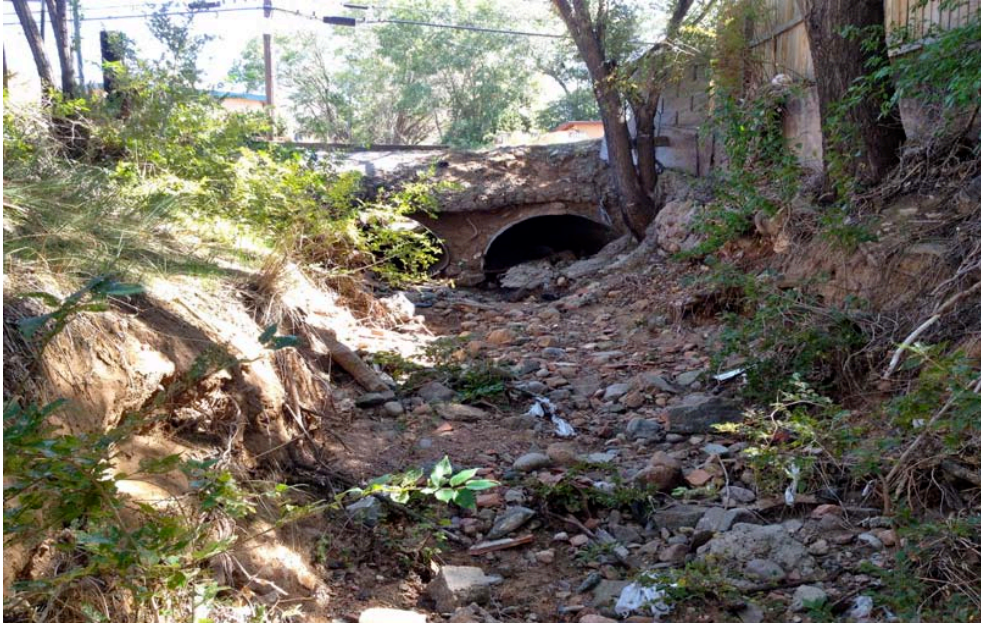
Culvert obstructed by cement dumped into Lower Arroyo Pinos, Segment B.
