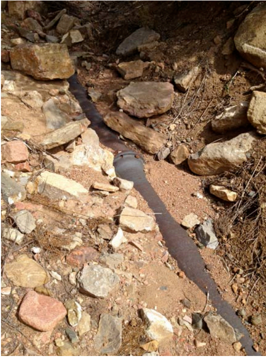
Exposed utility in Arroyo Piedra East, Segment A.
