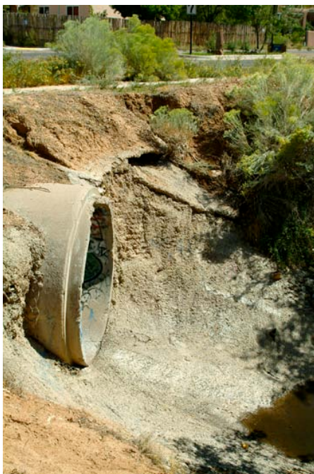
5 th street sidewalk threatened by erosion Lower Arroyo Pinos, Segment C.
