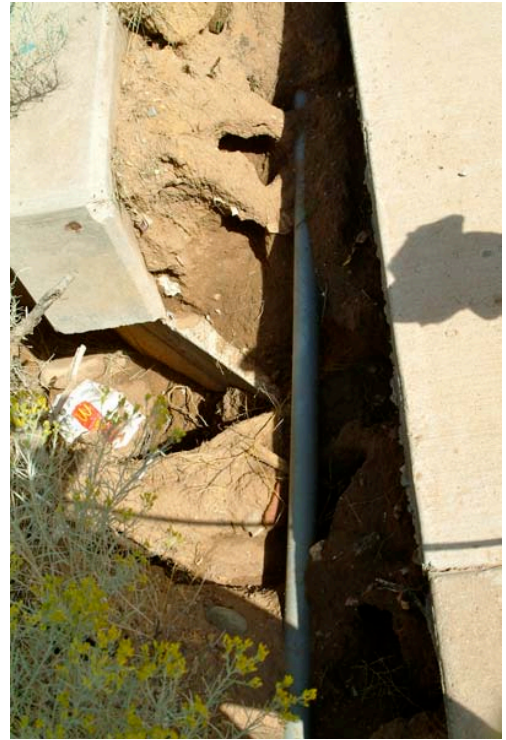
Exposed utility line off of Llano Street Bridge, Lower Arroyo Pinos, Segment C.
