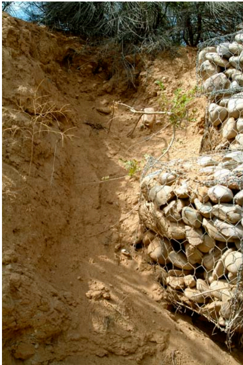
Erosion at edges of gabion walls, Lower Arroyo Pinos, Segment E.
