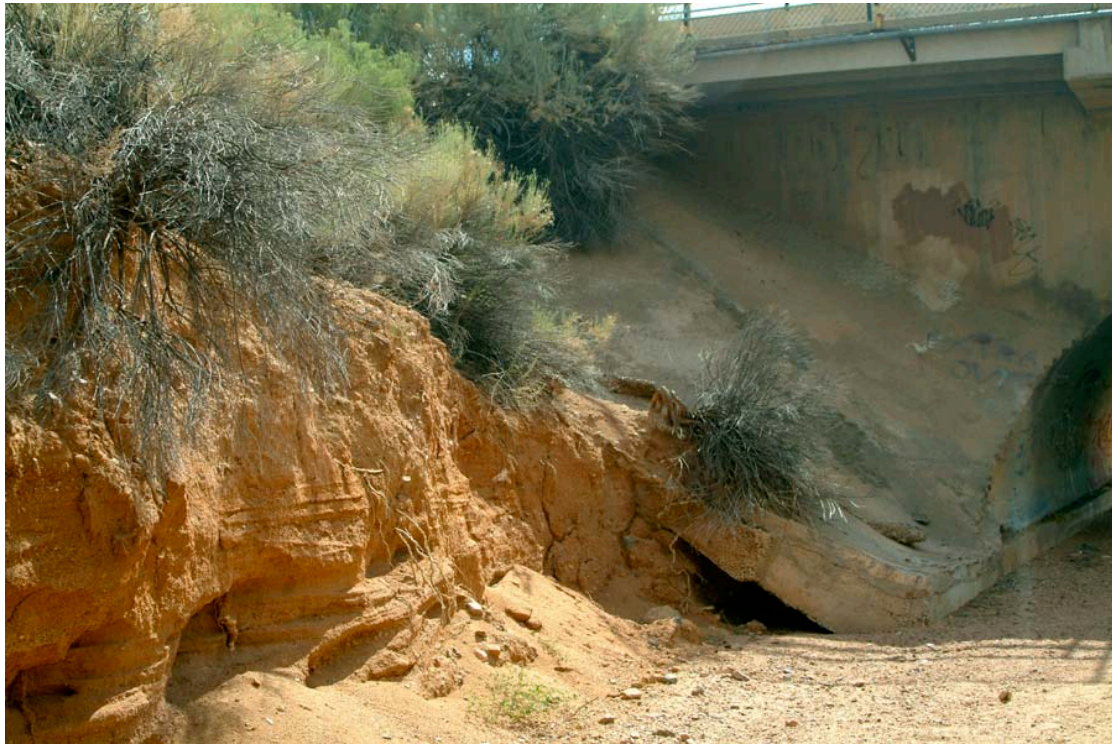
Erosion, collapsing banks and undercut bridge footings are a common sight in Segment D of the Arroyo de los Chamisos .
