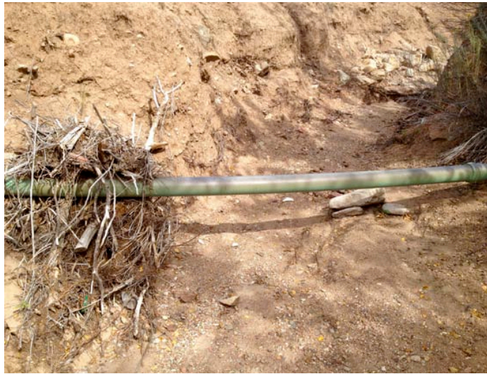
Exposed utility lines in Arroyo Piedra East, Segment A.
