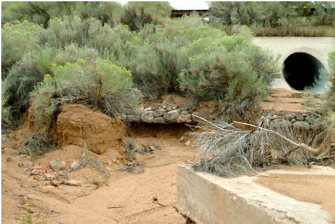
Erosion undercutting rip-rap, banks, and concrete outfall in Arroyo en Medio, Segment D.
