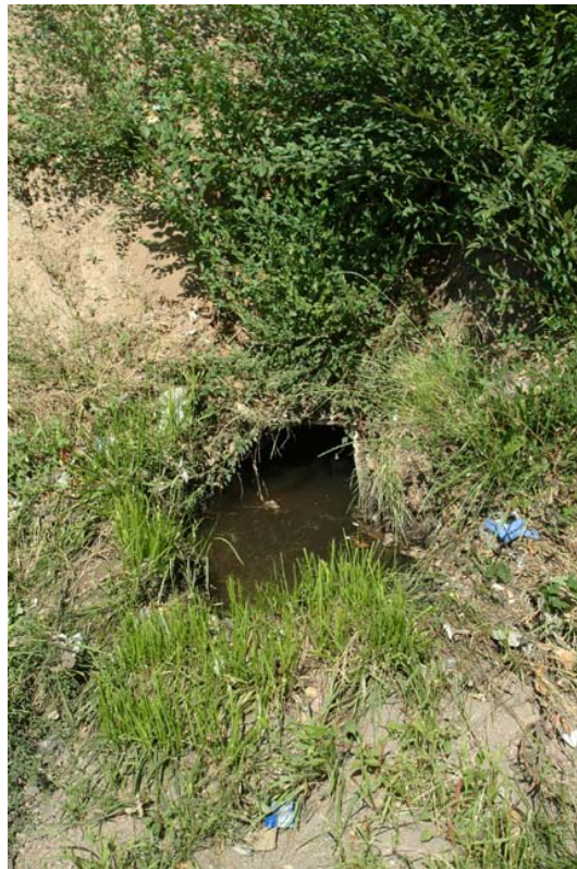
Clogged culvert, Lower Arroyo Pinos, Segment X.
