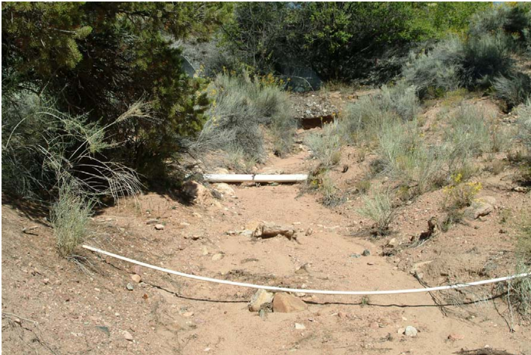
Exposed utility lines in the bed of Arroyo Piedra East, Segment B.
