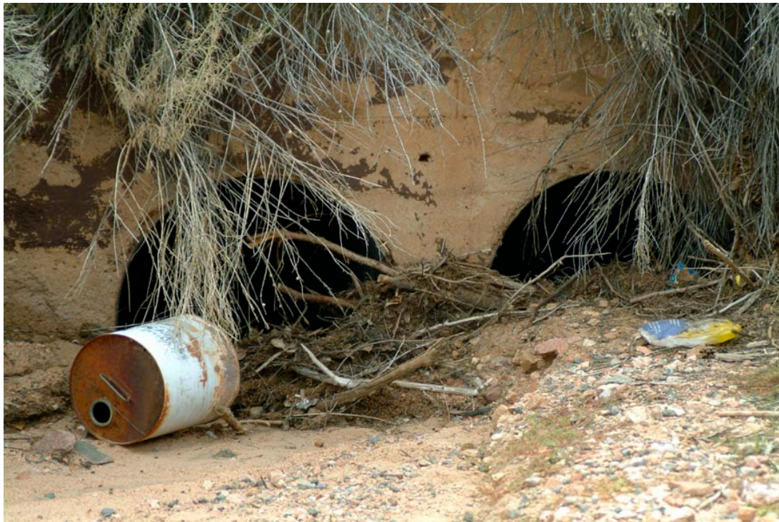
Obstructed culverts in Upper Arroyo Pinos, Segment B.
