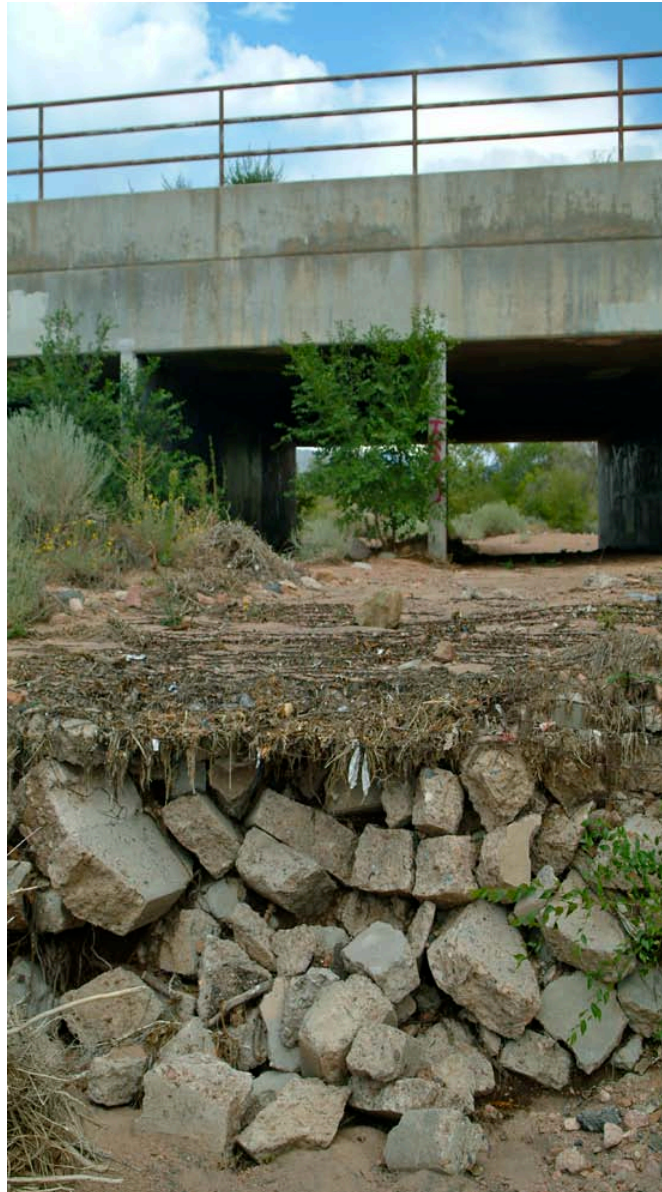
Rip – rap torn away from entire length of an outfall below Camino Carlos Rey Bridge crossing the Arroyo de los Chamisos in Segment F.
