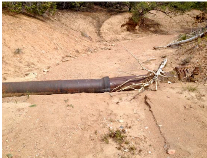
Exposed utility lines in Arroyo Piedra East, Segment A.
