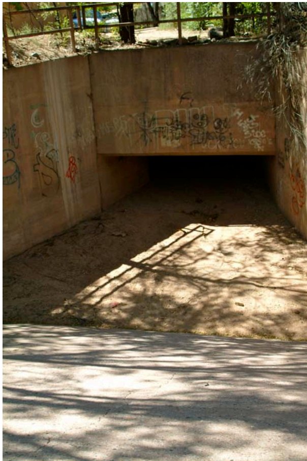
Box culvert trapping sediment beneath E. Alemeda Street, Arroyo Ancha Segment B.
