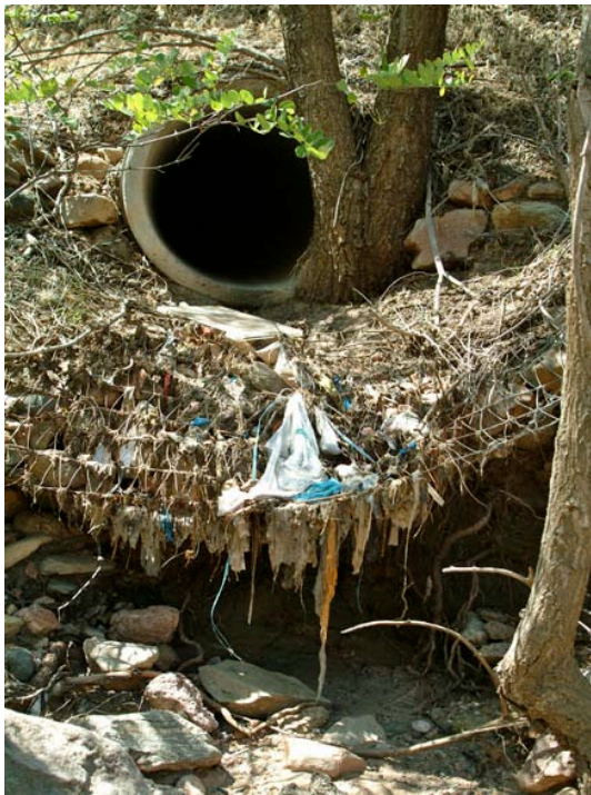
Damaged rip - rap with trash in Arroyo Cabra.
