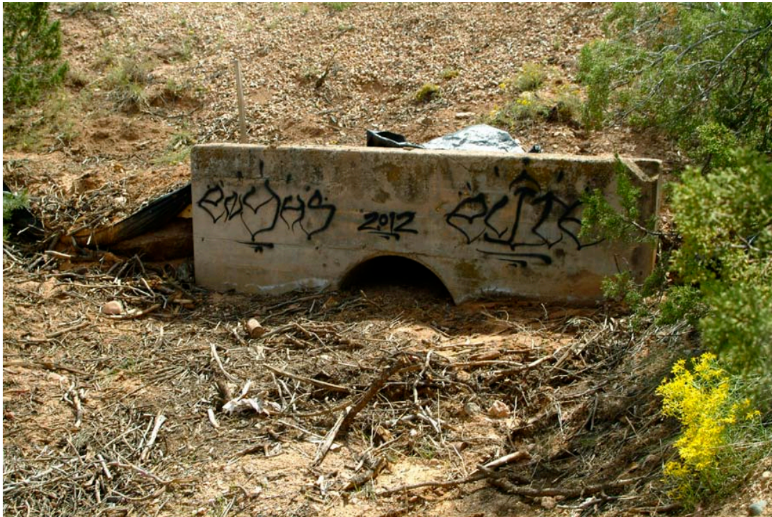
Plugged culvert near Old Pecos Trail in Arroyo Pinos, Segment A.
