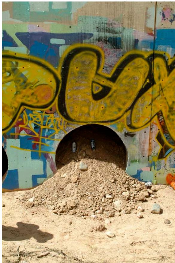
A clogged culvert at Old Pecos Trail, Upper Arroyo Pinos, Segment A.
