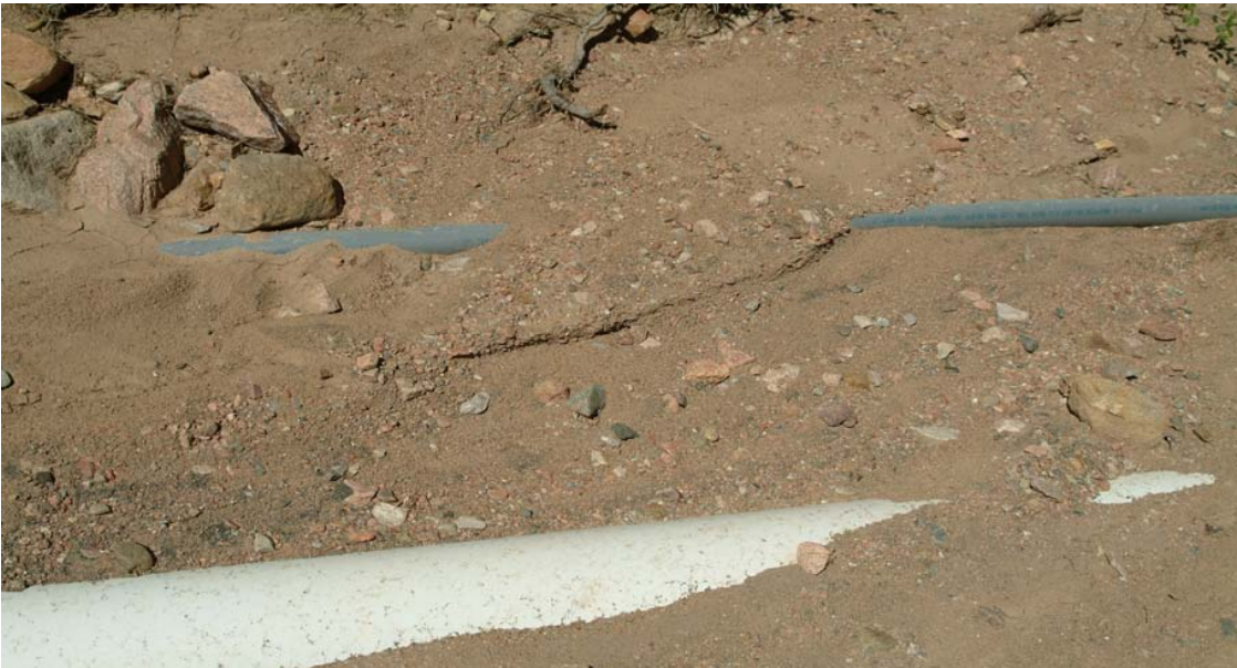
Two exposed pipes in Arroyo Ancha, Segment A.
