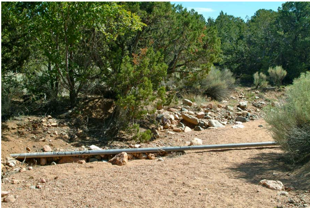
Exposed utility line in bed of Arroyo de los Chamisos, Segment A.
