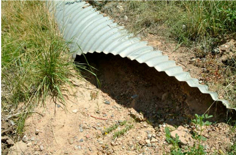
A silt clogged culvert in Arroyo Saiz.
