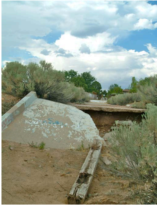
A broken outfall beside the Arroyo de los Chamisos Trail in Segment F.
