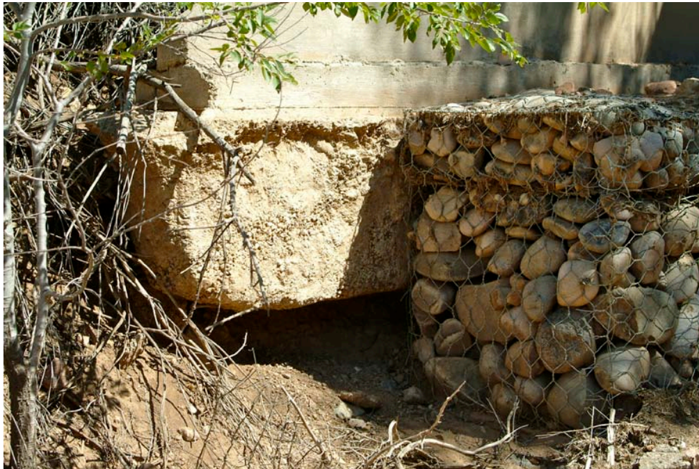
Undercut bridge footing in Arroyo Ancha, Segment B.
