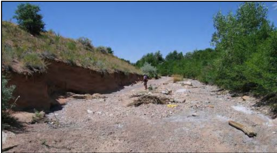
Figure 8.F. Undercut banks where design lacked reinforcement Photo facing downstream Source: photo by author (2005)
