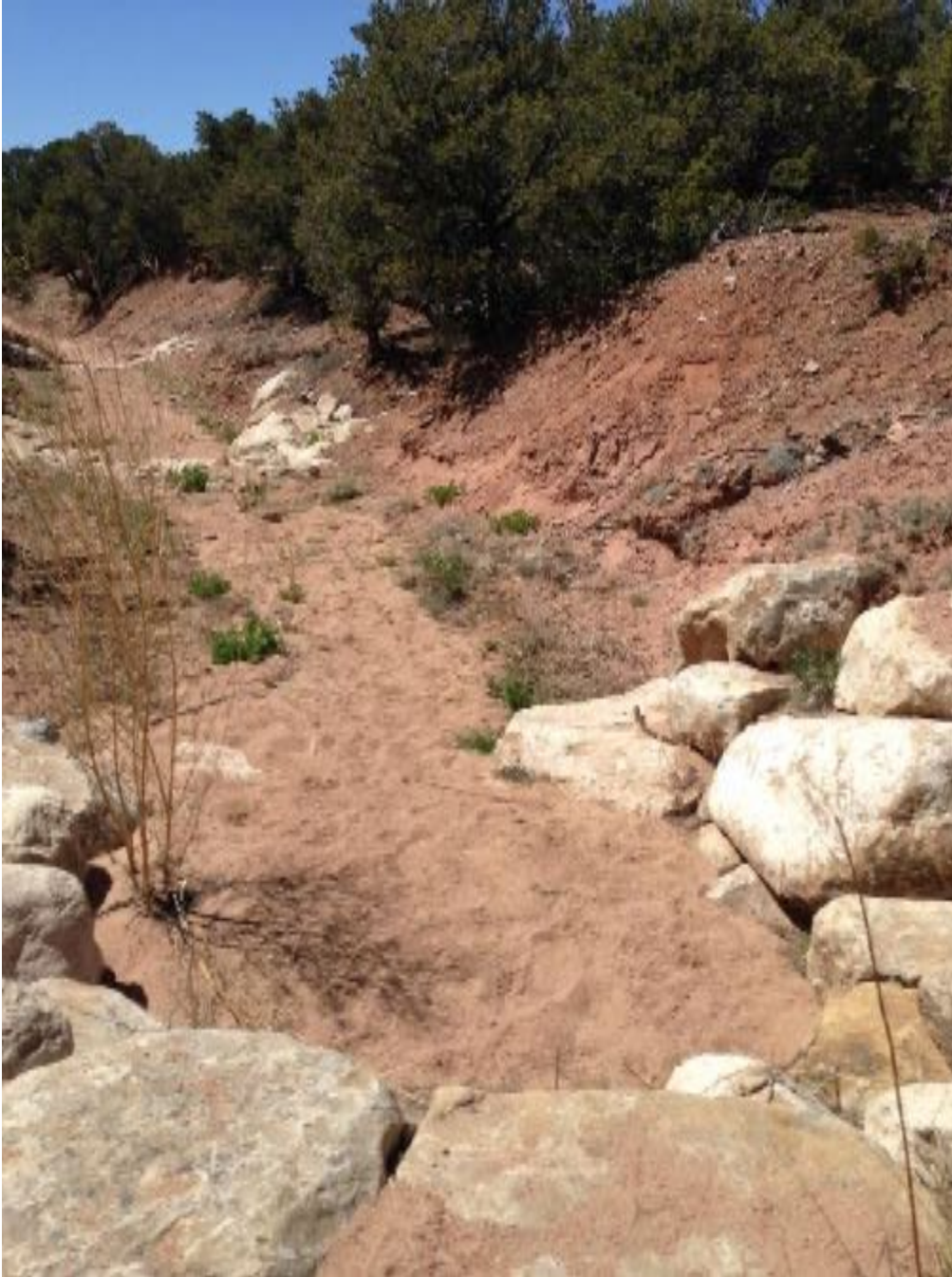
Segment A. One rock check dams, Upper Arroyo Pinos North, 2016.
