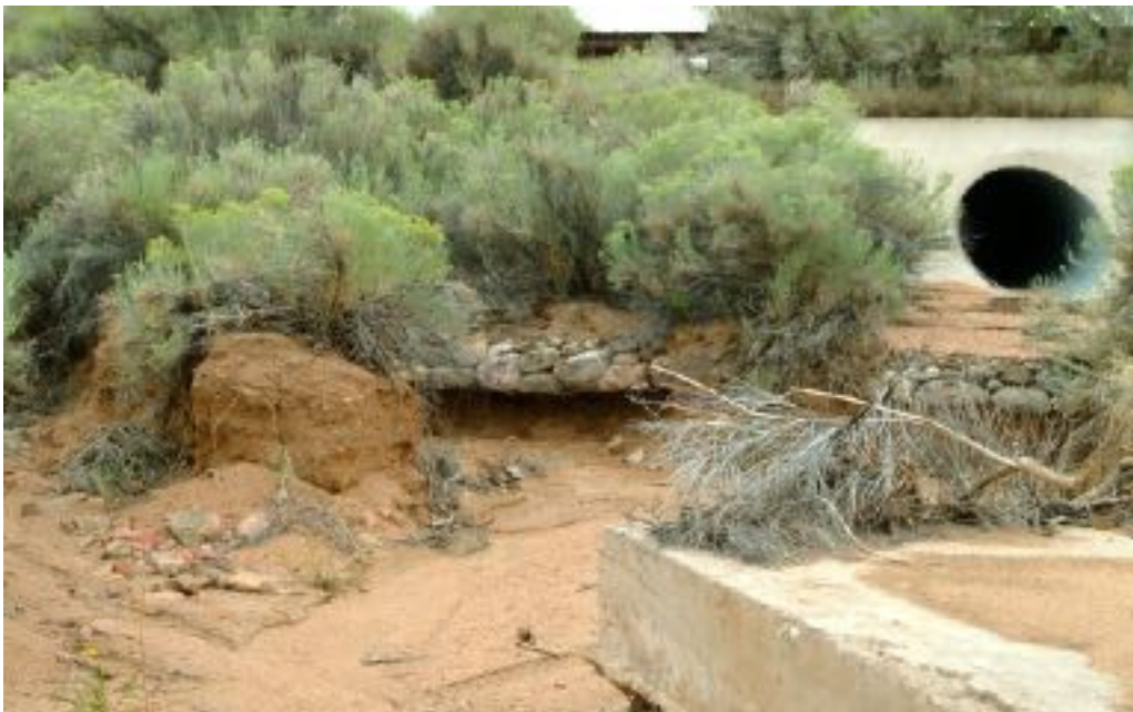
Segment D/ Example of one of many undercut rip rap, banks, in Arroyo en Medio, 2012.
