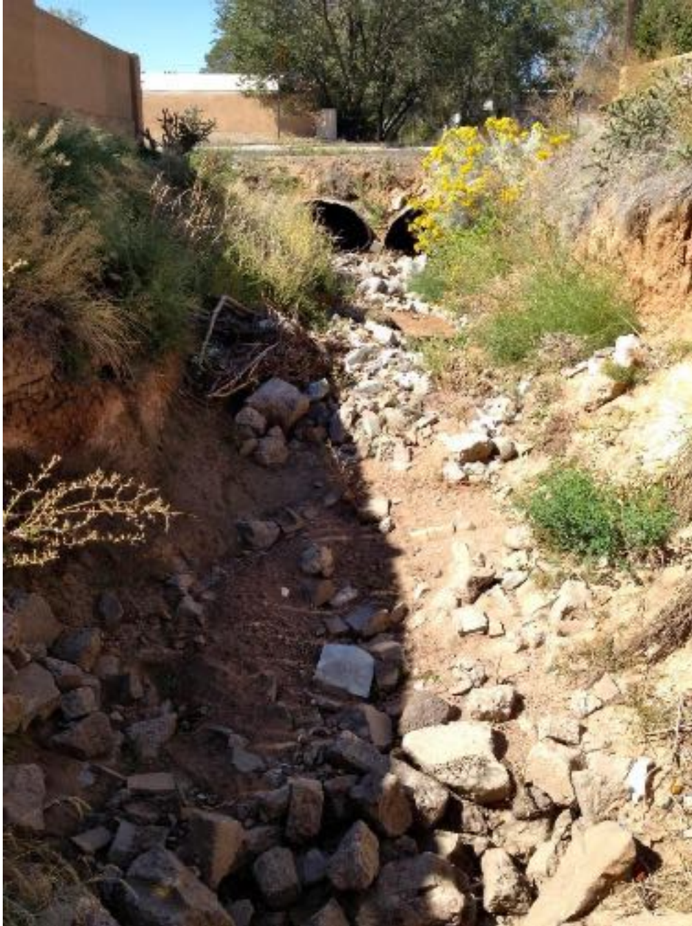
Segment B /Bank erosion below private property, Lower Arroyo Pinos, 2012.
