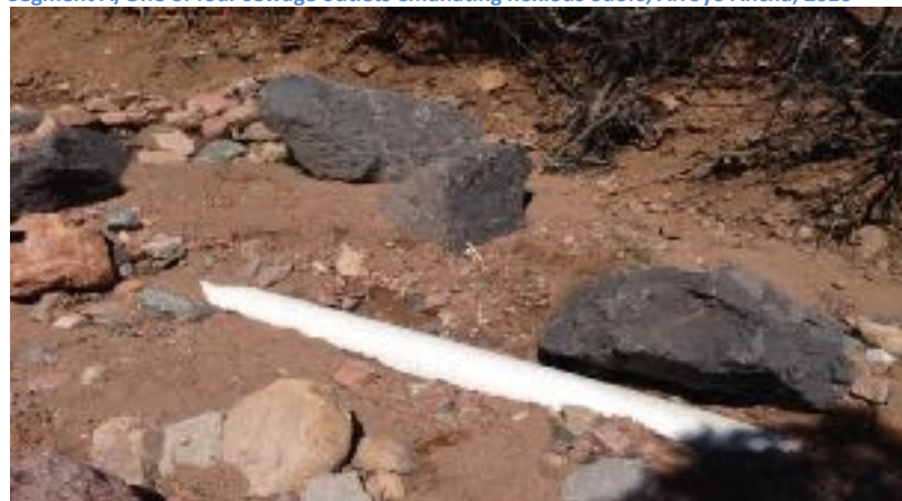
Segment A/ Exposed sewer line in Arroyo Ancha, 2016
