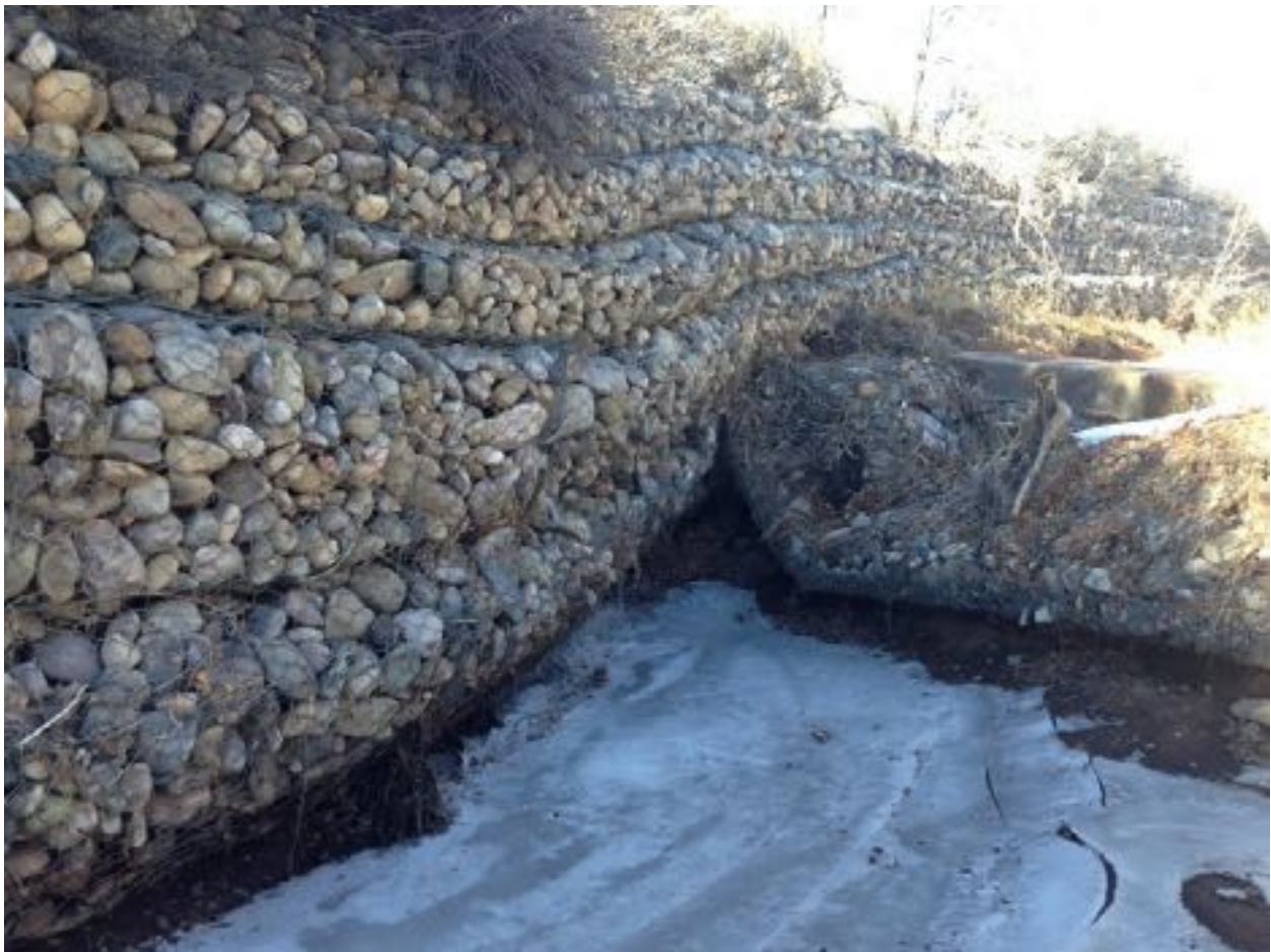
Segment C/, Gabion walls sagging, Lower Arroyo Pinos, 2016.
