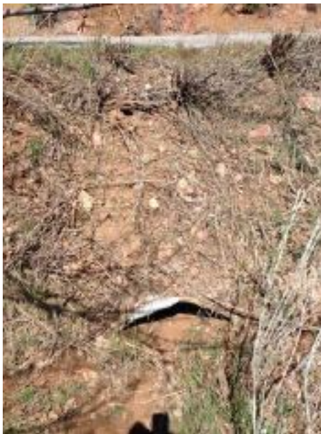
Segment A/Obstructed culvert, Arroyo Ancha, 2016
