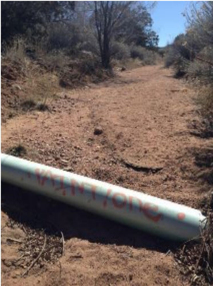
Segment G/Disconnected storm culvert in Arroyo en Medio ,2016.
