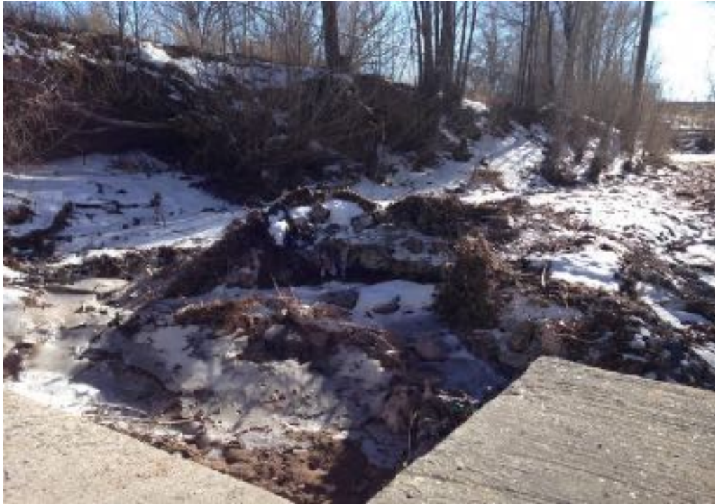
Segment D/ Damaged rip rap mat 2016, Lower Arroyo Pinos.
