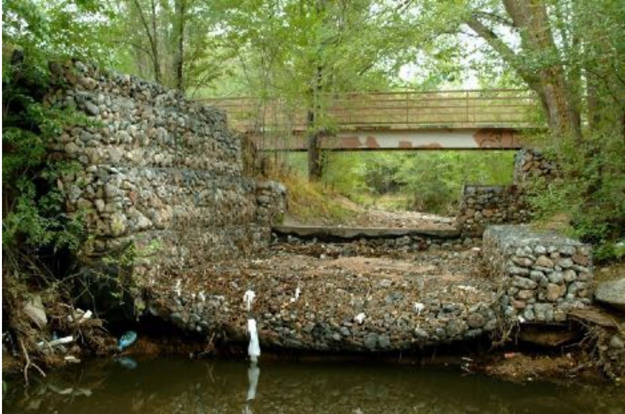
Segment C/ Water standing in deep scour below undercut rip rap mat, Lower Arroyo Pinos, 2016.
