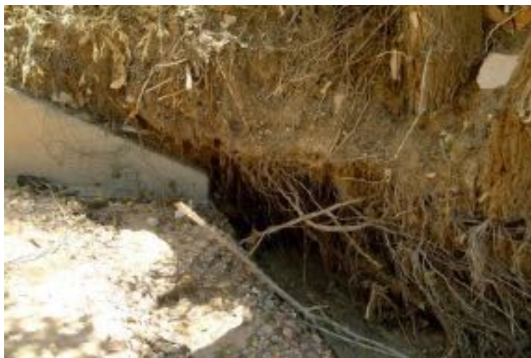
Segment B/ Bank erosion by check dam, Arroyo Ancha, 2016
