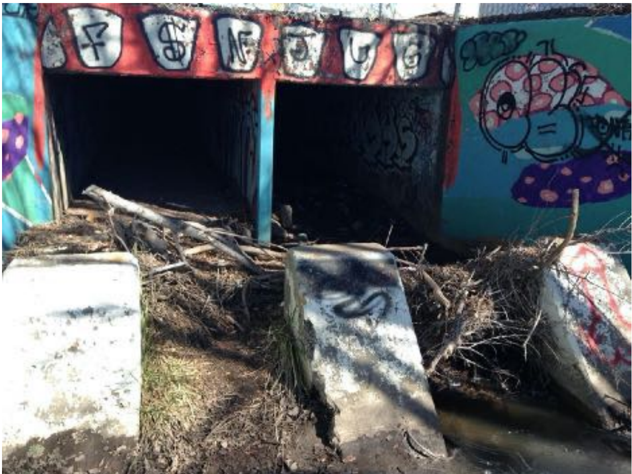
Segment X/ Debris caught in storm outlet , Lower Arroyo Pinos, 2016.
