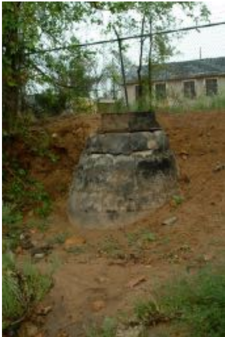
Segment E/ Unprotected Sewer utility, Lower Arroyo Pinos, 2012.
