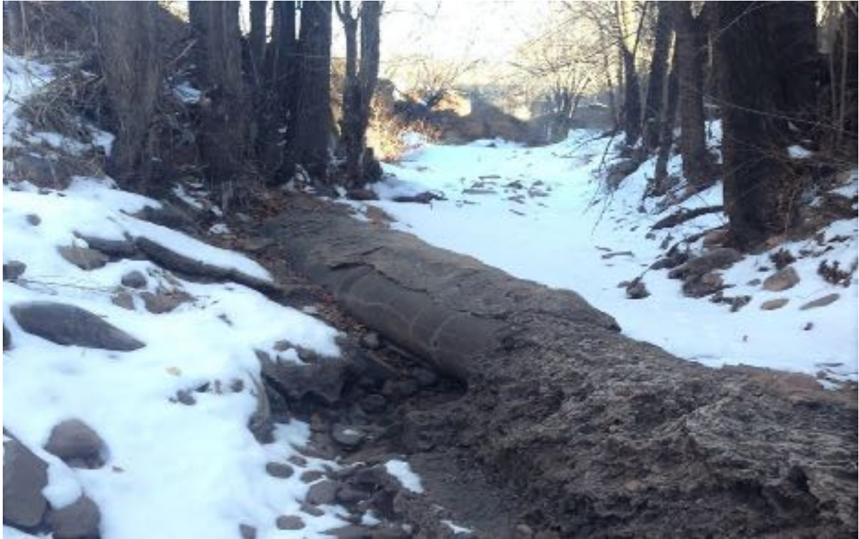
Segment C/Cracked concrete pipeline, Lower Arroyo Pinos, 2016.
