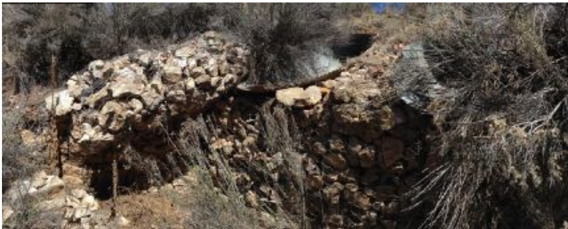
Segment A/Gabion askew, Arroyo Ancha, 2016.
