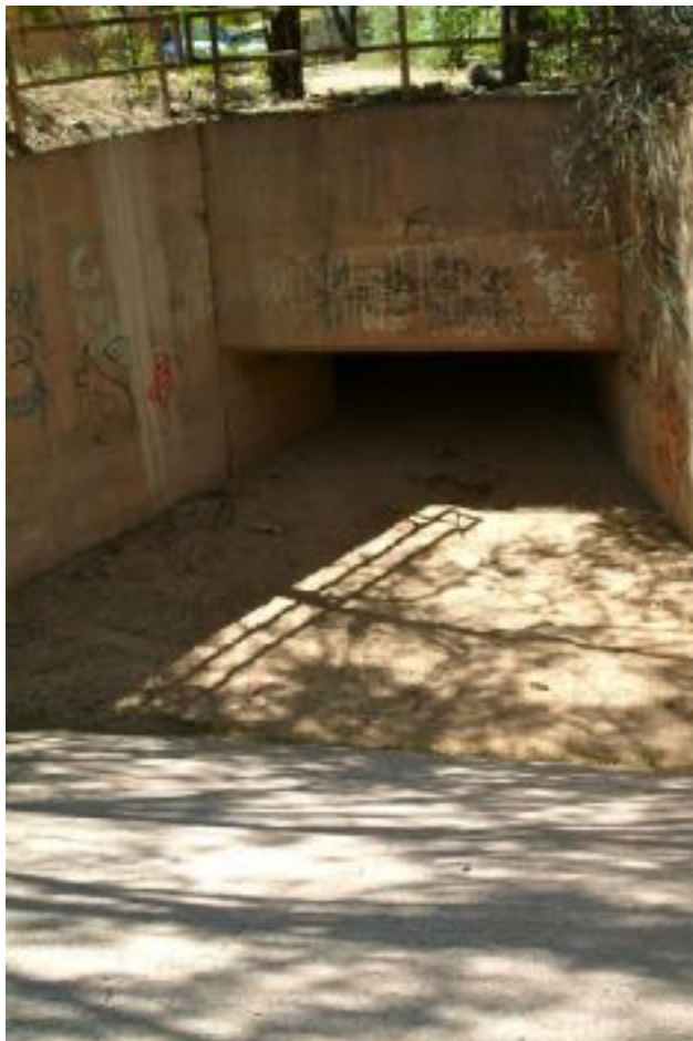
Segment B/ Box culvert trapping sediment beneath E. Alameda St., Arroyo Ancha, 2012.
