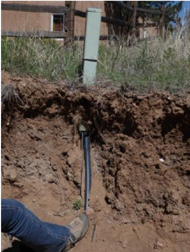
Segment A/Exposed cable, Arroyo Cloudstone, 2016.
