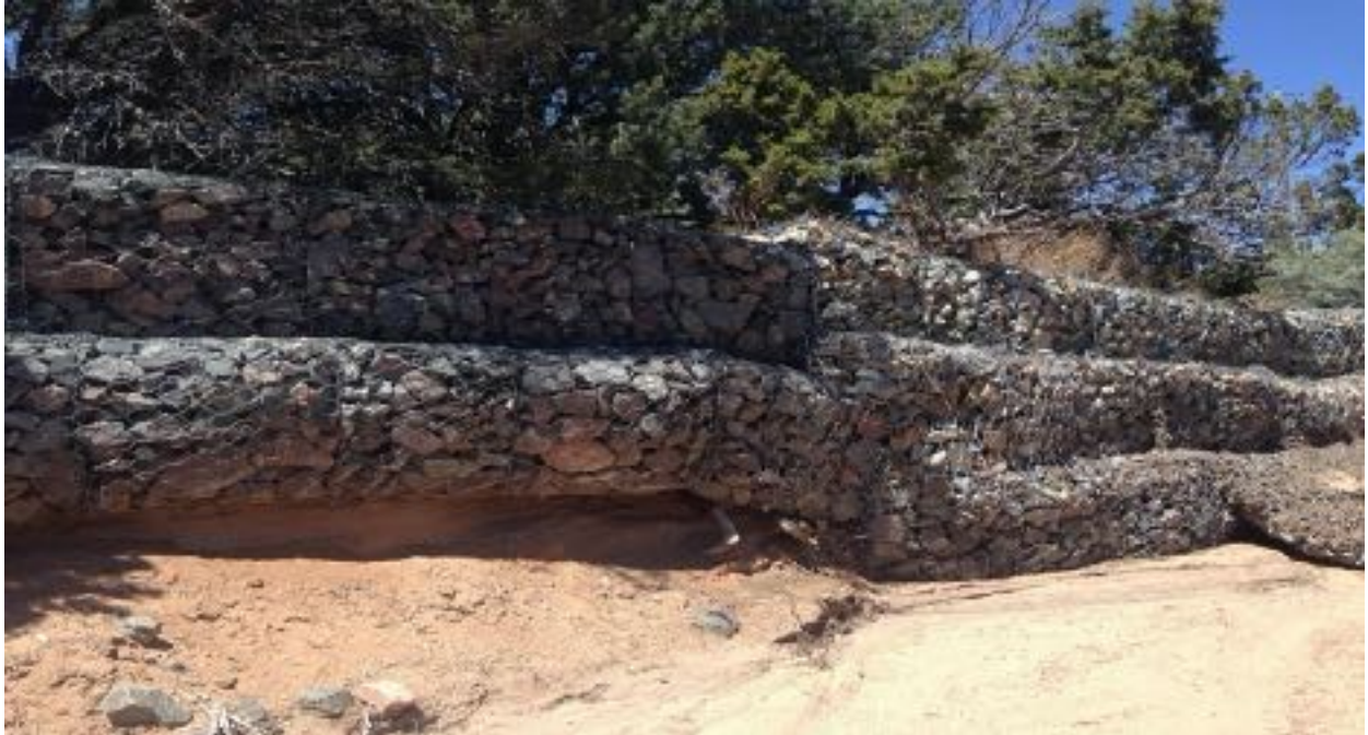
Segment B/Erosion below gabion walls, Arroyo Cloudstone, 2016.
