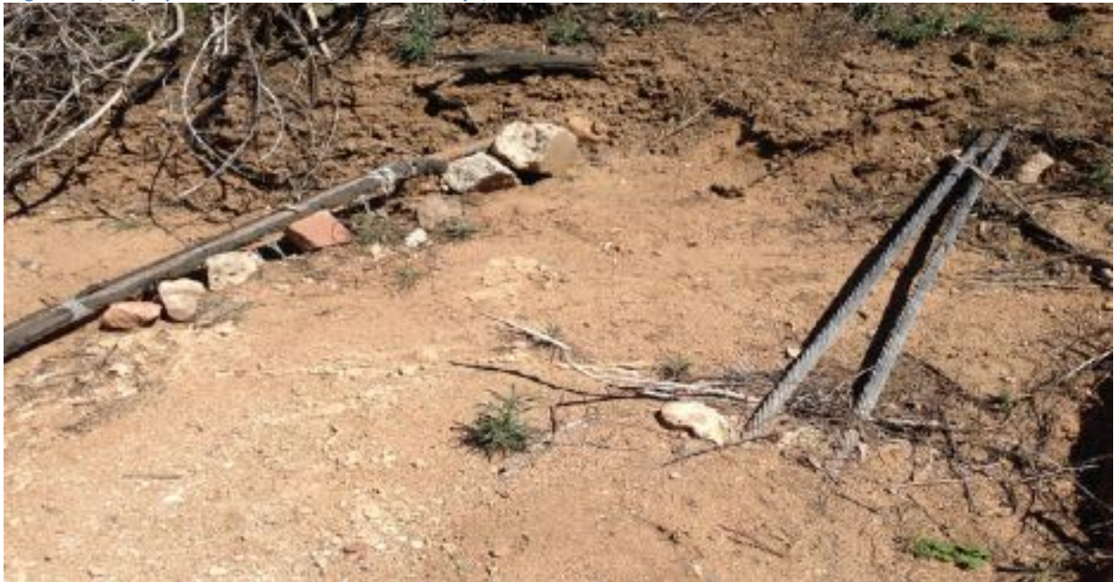
Segment A/ Exposed cables, Foothills Arroyo, 2016.
