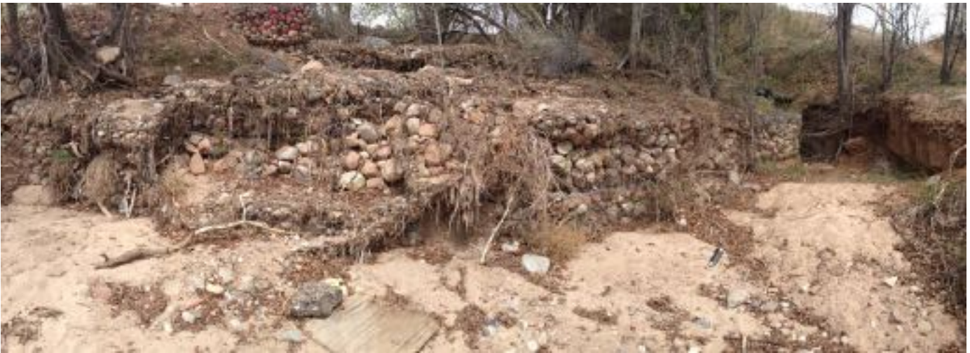
Segment B/Collapsing gabion and bank collapse (far right), Arroyo Torreon, 2016.
