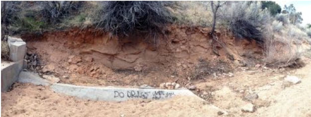
Segment B/ Bank deterioration at check dam, Arroyo Chaparral ,2016.
