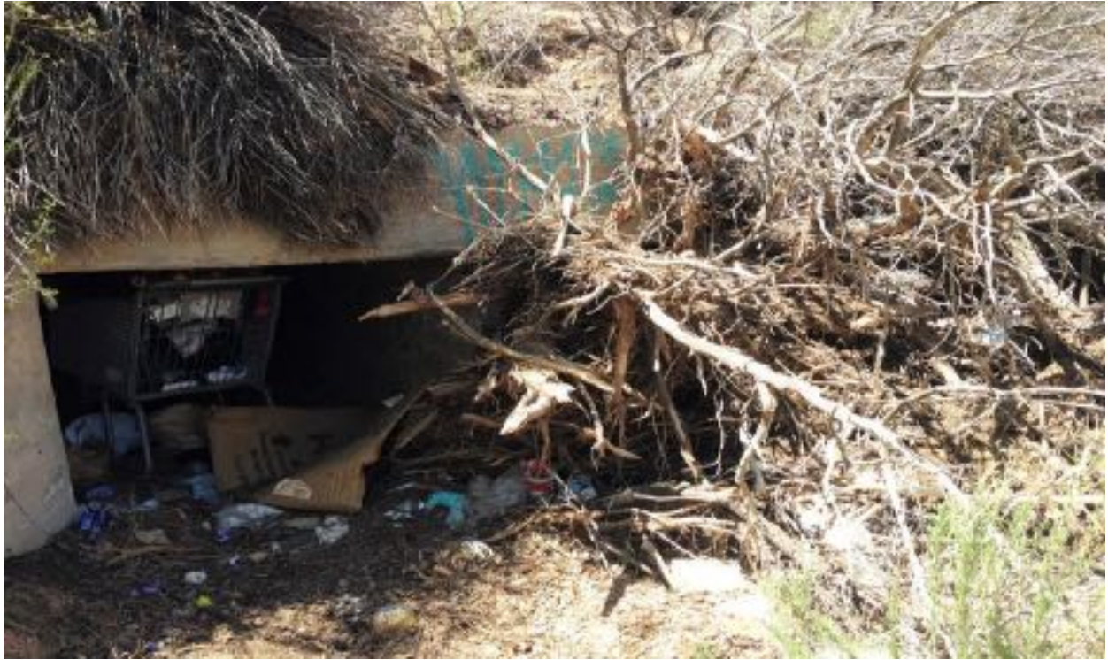
Segment A/ Obstructed box culvert with transient camp, Foothills Arroyo, 2016.
