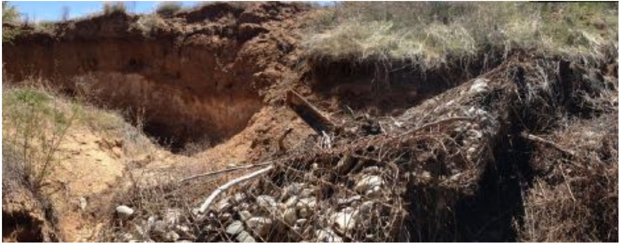
Segment A/ Vertical walls with rip rap mat folded back from flooding, Foothills Arroyo, 2016.
