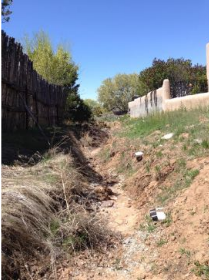
Segment A/ Drain pipes protrude into arroyo from private property, Foothills Arroyo, 2016.
