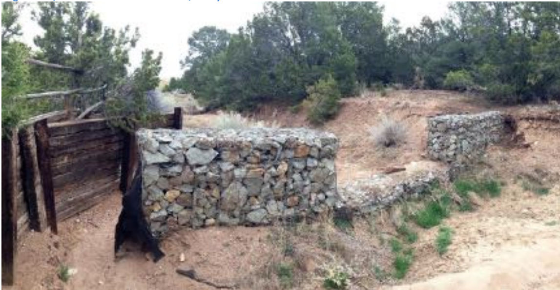
Segment B/ Same gabion check dam with added retaining wall, Arroyo Piedra, 2016
