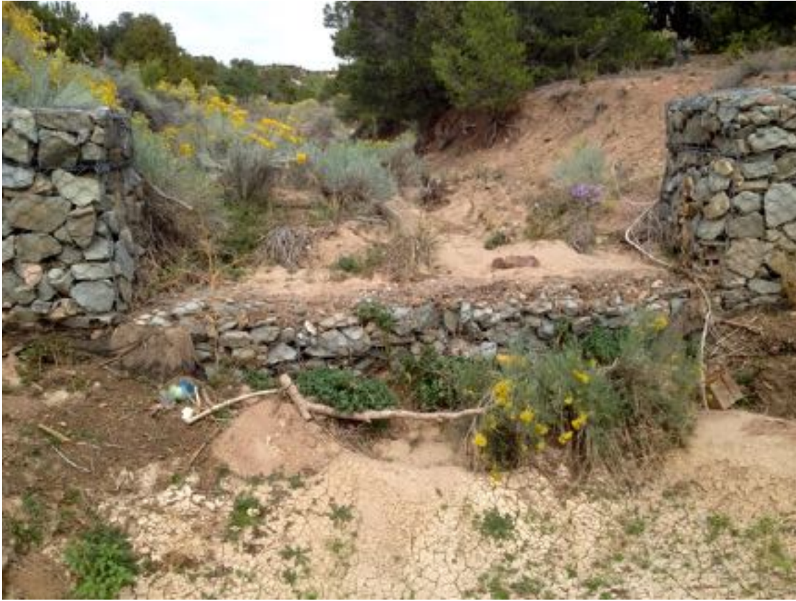
Segment B/ Gabion check dam in 2012, Arroyo Piedra.
