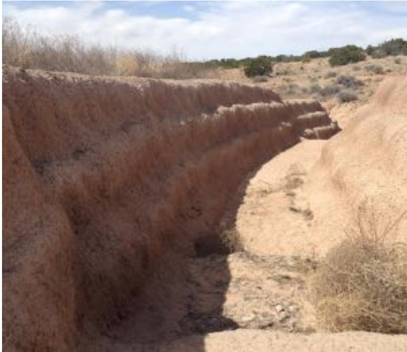
Segment B/Two views of engineered walls made of tire and adobe with undercutting, Arroyo Torreon, 2016.
