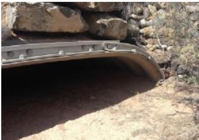
Segment A/Silt trapped in culvert, Arroyo Torreon, 2016.
