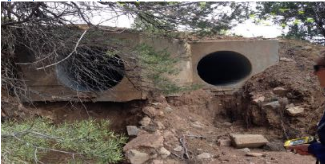
Segment B/Bank deterioration below culverts, Arroyo Piedra, 2016.
