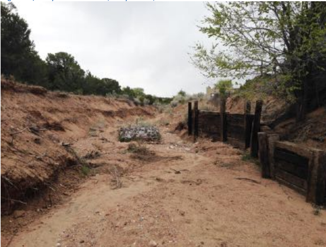
Segment B/ Retaining wall and gabion basket added to arroyo channel, Arroyo Piedra, 2016
