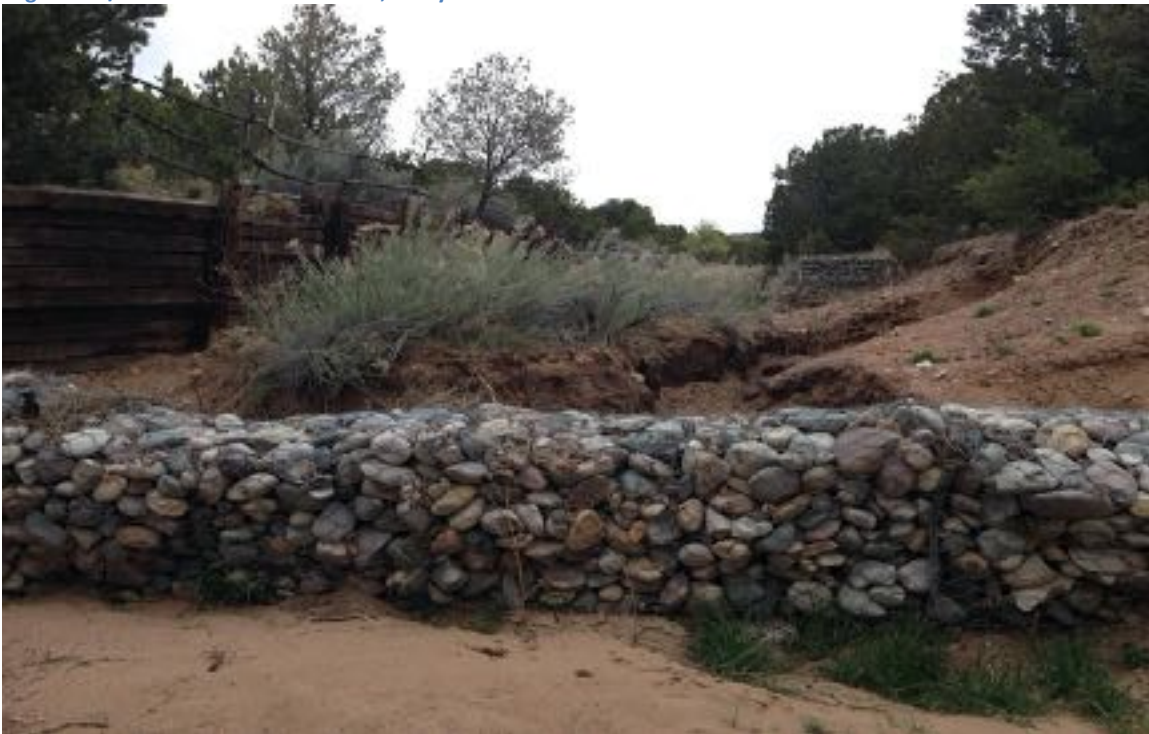
Segment B/ Same gabion check dam with added retaining wall, Arroyo Piedra, 2016
