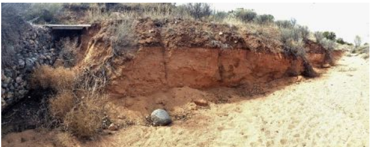
Segment B/ Bank deterioration at gabion wall check dam, Arroyo Chaparral ,2016
