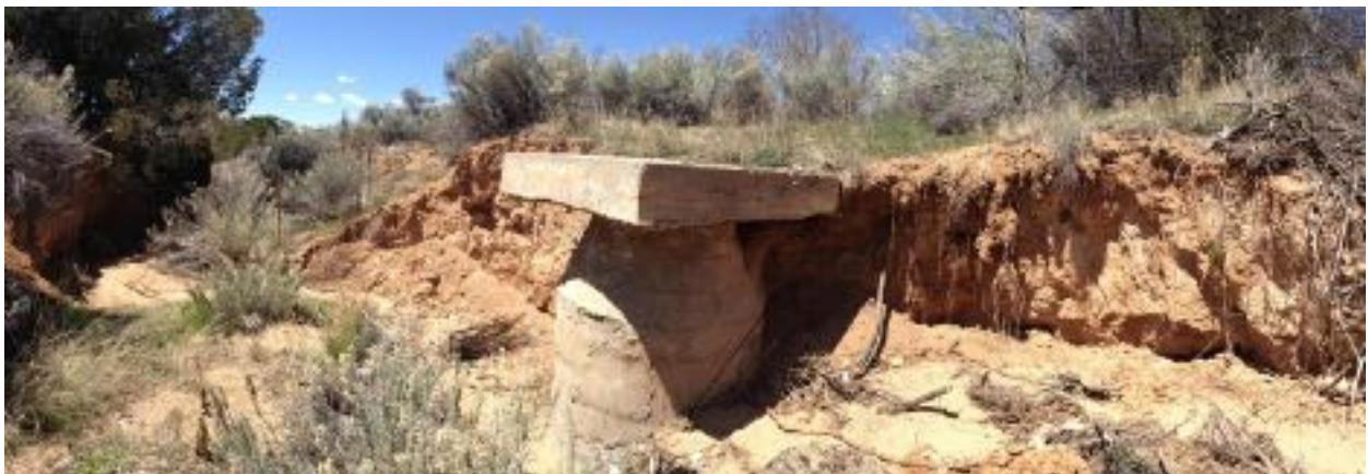
Segment A/ Exposed cables, deteriorating banks and sewer outlet, Foothills Arroyo, 2016.
