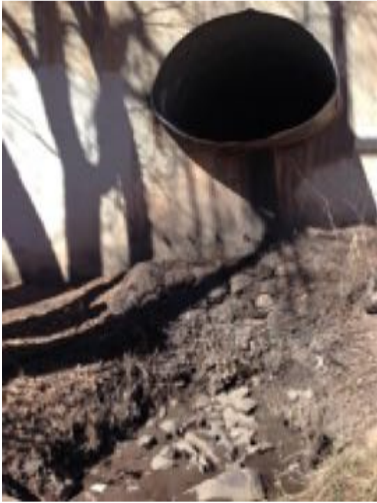
Segment D/Comparison of rip rap damage below culvert, Arroyo Mascaras , 2016.
