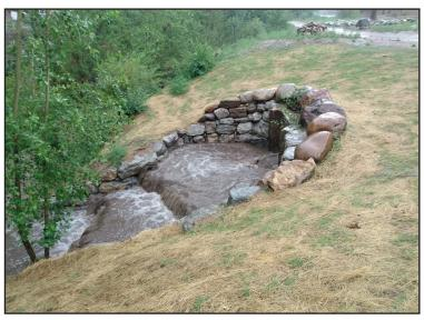
Our completed Zuni Bowl at the end of Camino Escondido slows stormwater runoff and protects the riverbank from erosion.
